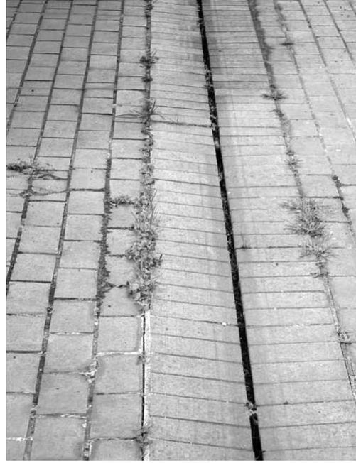
Plants in mortar joints on Cromwell Highwalk
