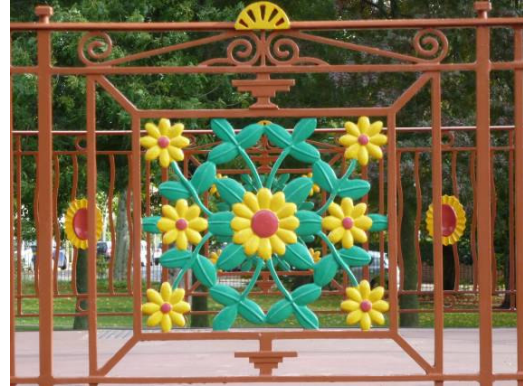
Detail of balustrade
