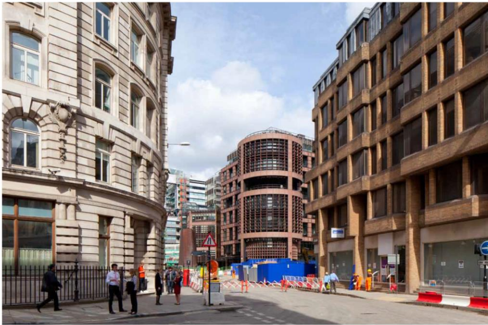
Existing view from junction of Finsbury Circus and Blomfield Street looking north-east
