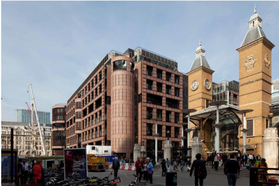
Existing view from Liverpool Street looking north-west
