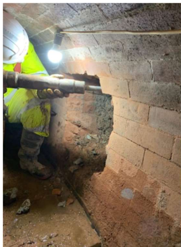
Devonshire Row Sewer – Repairing a collapsed connection
