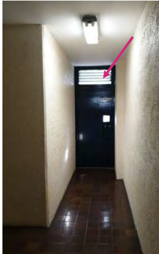
Figure 17: Stair/lift lobby vent (red arrow) for Staircase 24
