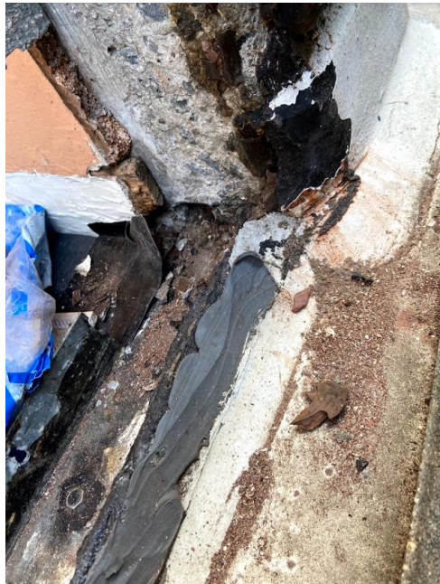
Figure 16: Aperture of a balcony door frame showing no cavity
