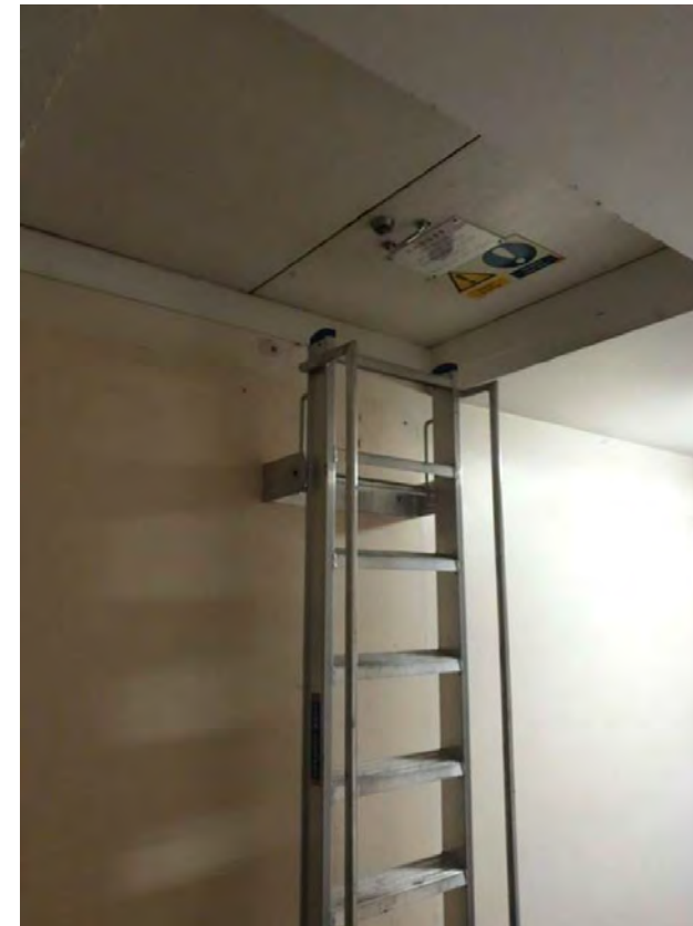
Figure 6: Fixed ladder to plant area in L7 Staircase 26
