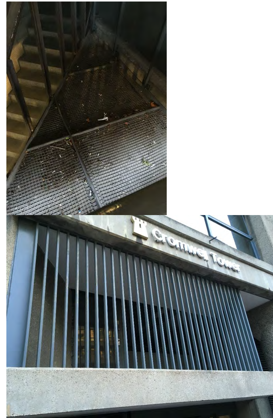
Figure 25: Permanent opening at the bottom of the firefighting stair at Podium Level
