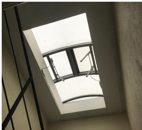
Figure 22: Staircase 49 opening vent
