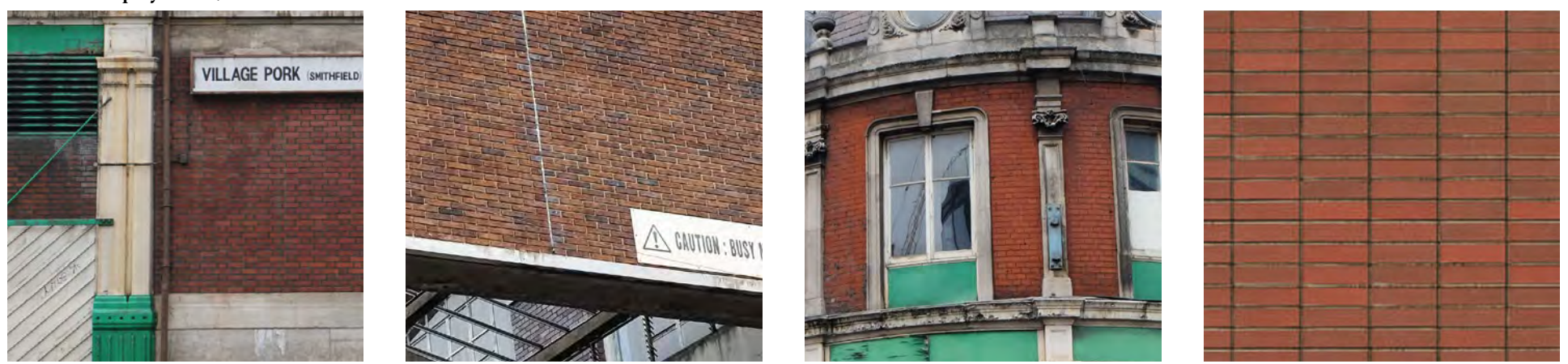
Original Course: Flemish bond Secondary Course: Running Bond Tertiary Course: English Bond New Infill: Stacked bond red brickwork
