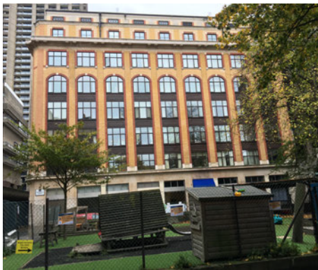
Bridgewater House northern elevation
