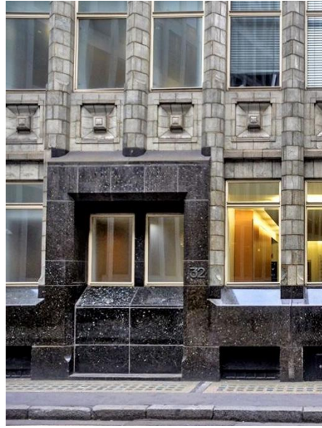
View 2: Entrance to No. 32 currently blocked
