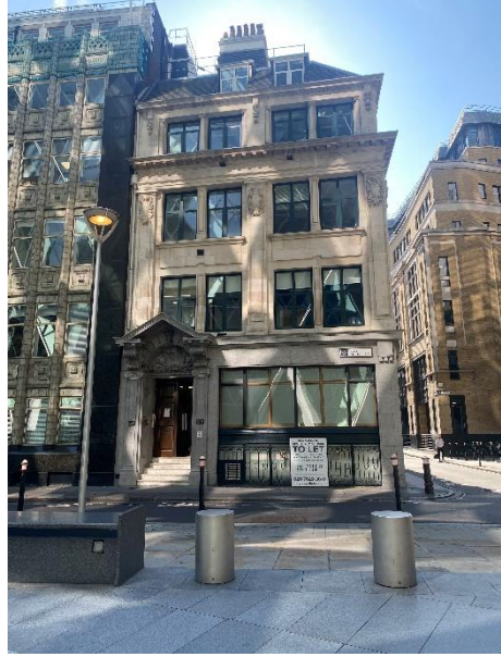
View 2: Bury Street (facing St. Mary Axe)
