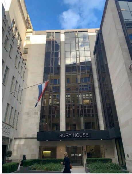
View 2: Bury Street
