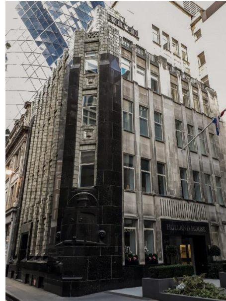
View 3: Bury Street (Holland House Main Entrance)
