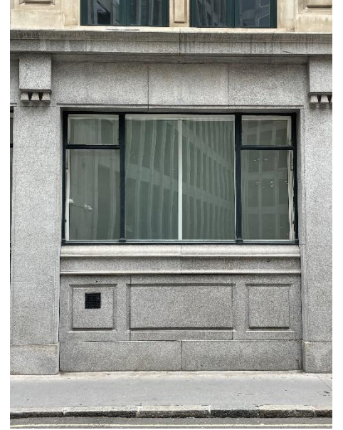
View 4: Bury Street
