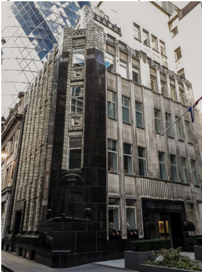
Figure 2: View of Holland House (southwest elevation) from Bury Street.
