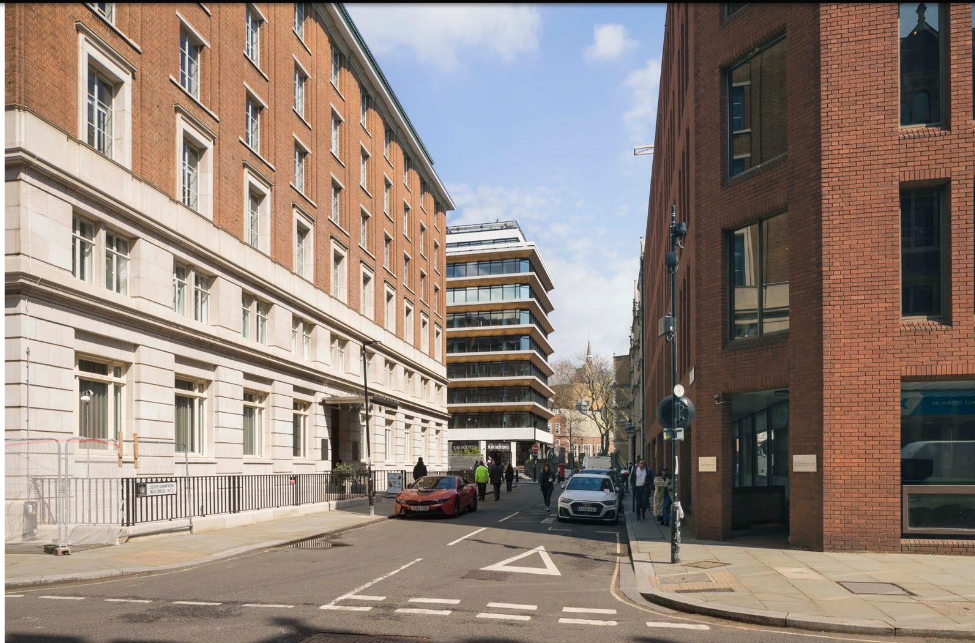
Existing view – Chancery Lane
