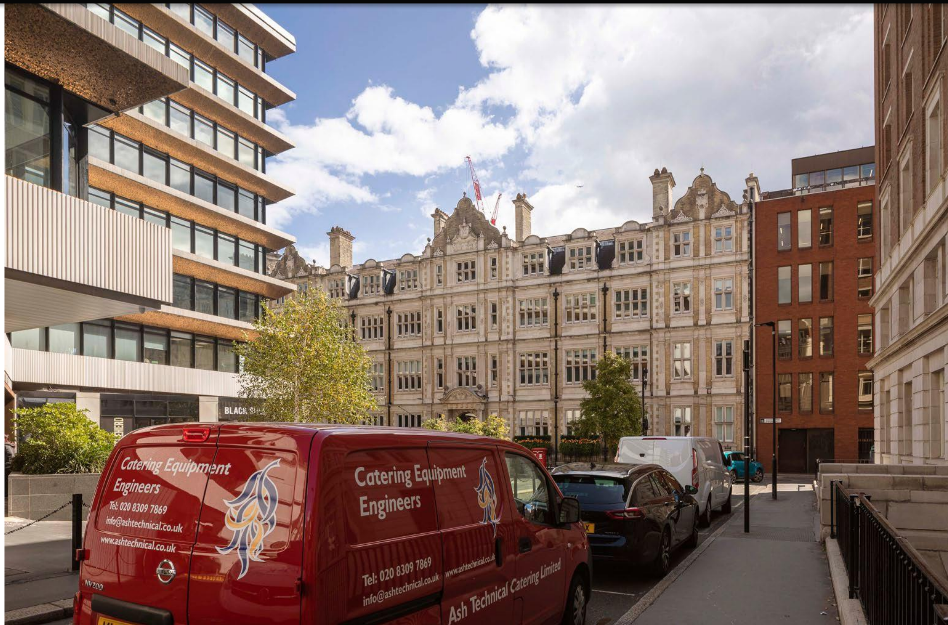
Existing view - Southampton Buildings, south
