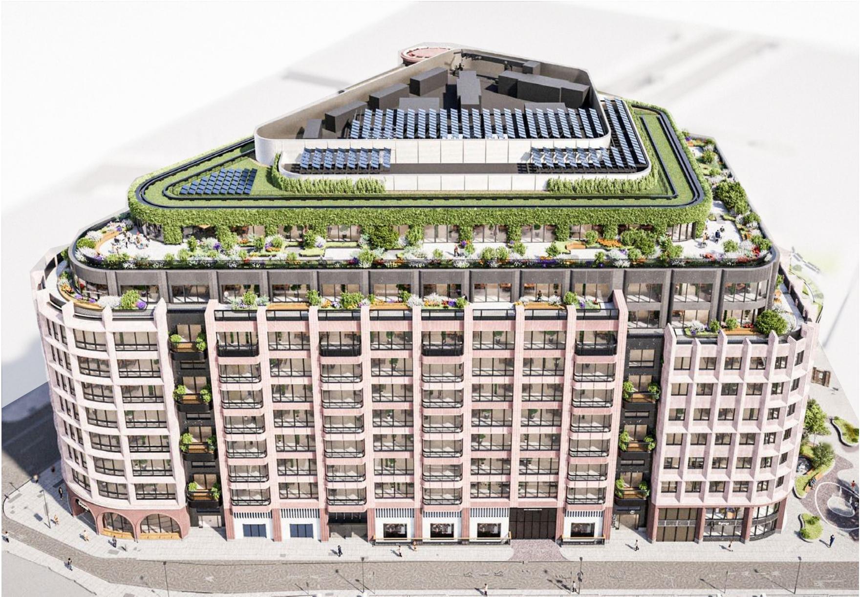
Building envelope and appearance - Roof (fifth elevation)
