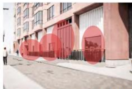
Location 3: Art Vitrines and Loading Bay Door
