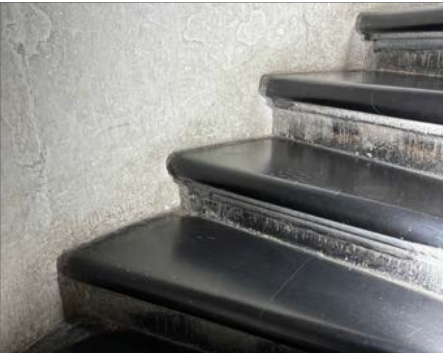
Fig. 34 Black limestone indents to stair treads, 2024
