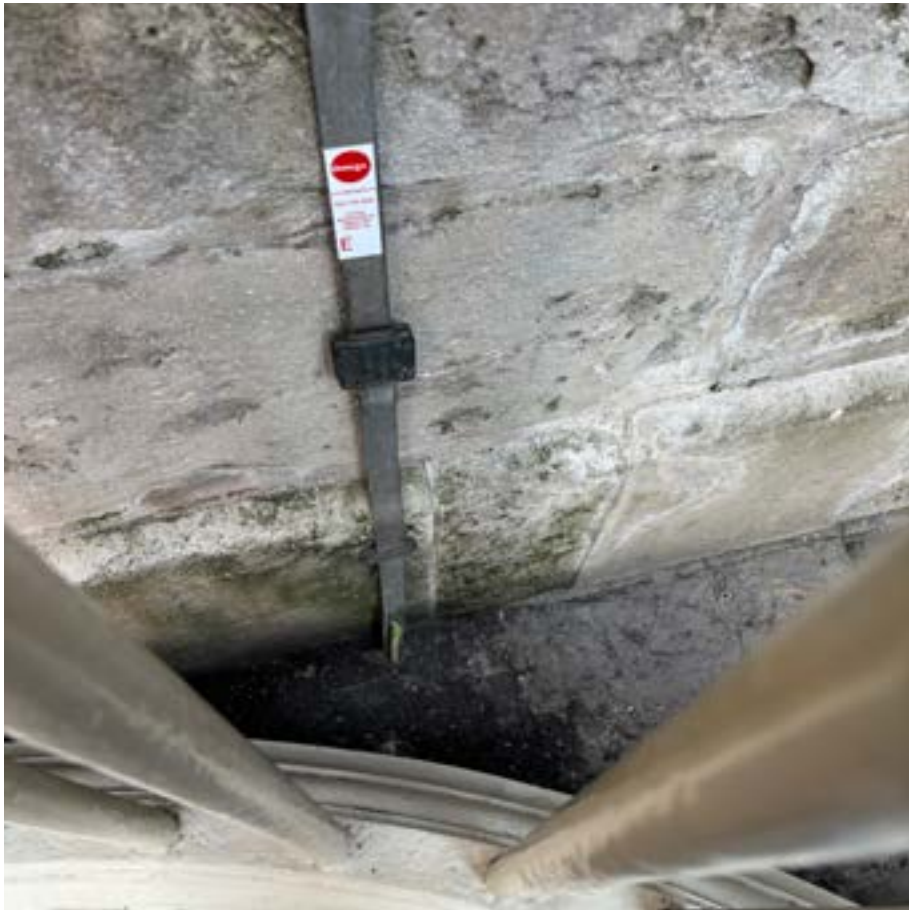
Fig. 80 Exterior lightning protection tape, 2024
