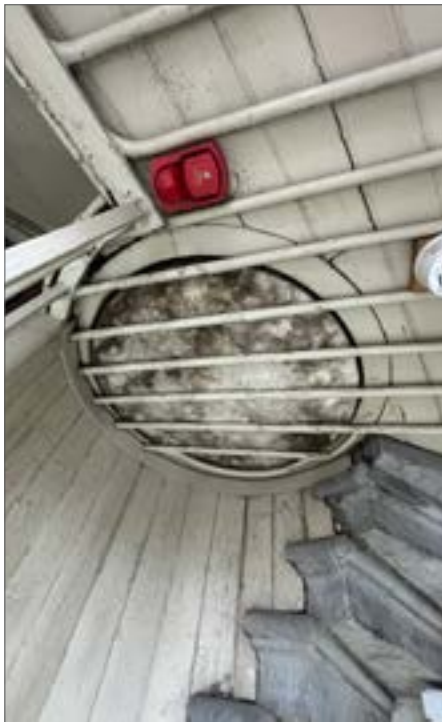
Fig. 49 Steel flat clasped to balusters, 2024
