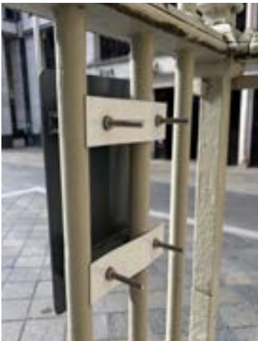
Fig. 108 Crude fixings to CoL sign, 2024
