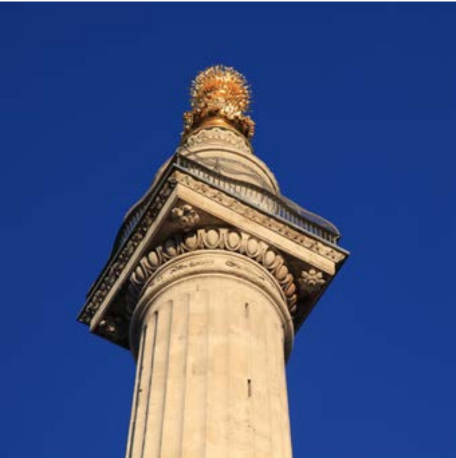
Fig. 76 Carved stone paterae on the underside of the column abacus, 2009
