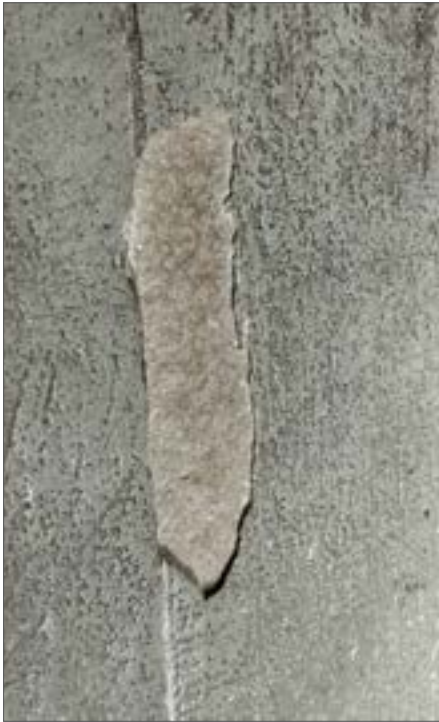
Fig. 33 Local spalling of stonework, 2024
