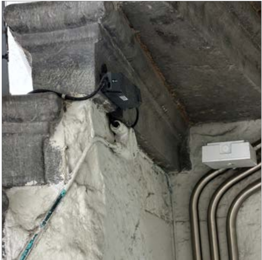
Fig. 101 White emergency light and black transformer, 2024
