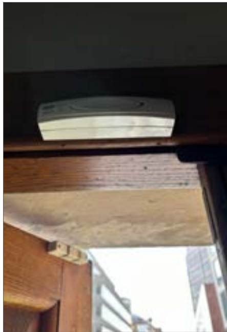
Fig. 27 Door movement detector, 2024
