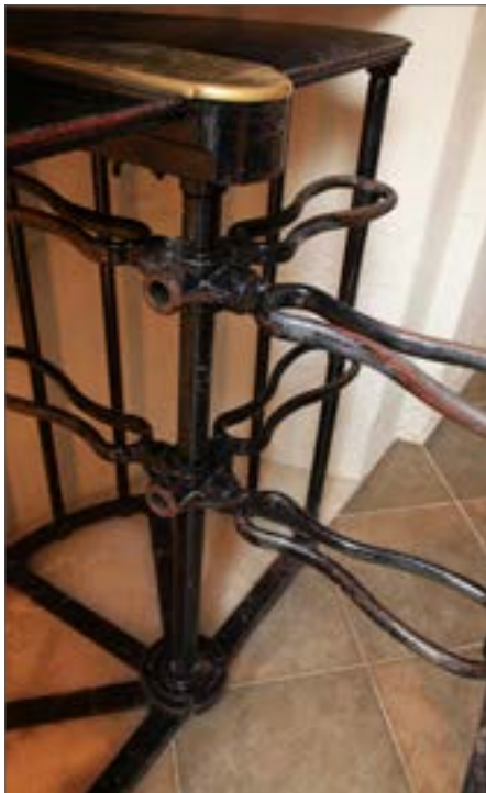
Fig. 68 Turnstile shown open, (one set of arms is missing), 2024
