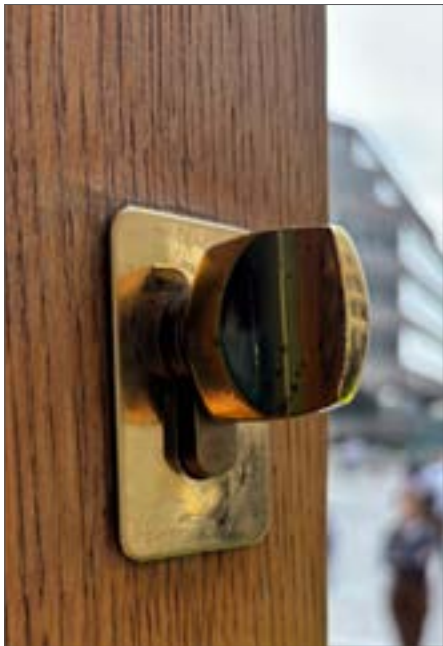
Fig. 25 Mortice escape latch, 2024
