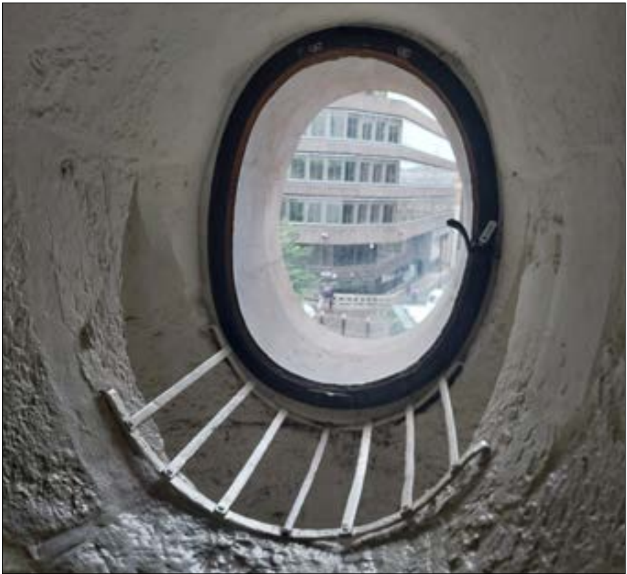
Fig. 54 Iron oval casement window, 2024
