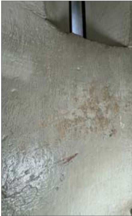
Fig. 32 Eroded paintwork, 2024
