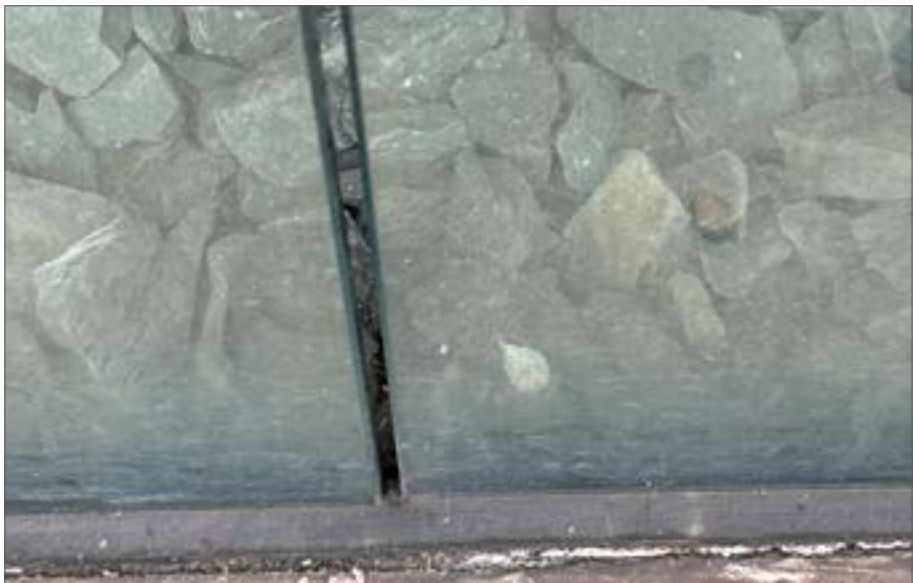
Fig. 120 Open joints between structural glass, 2024
