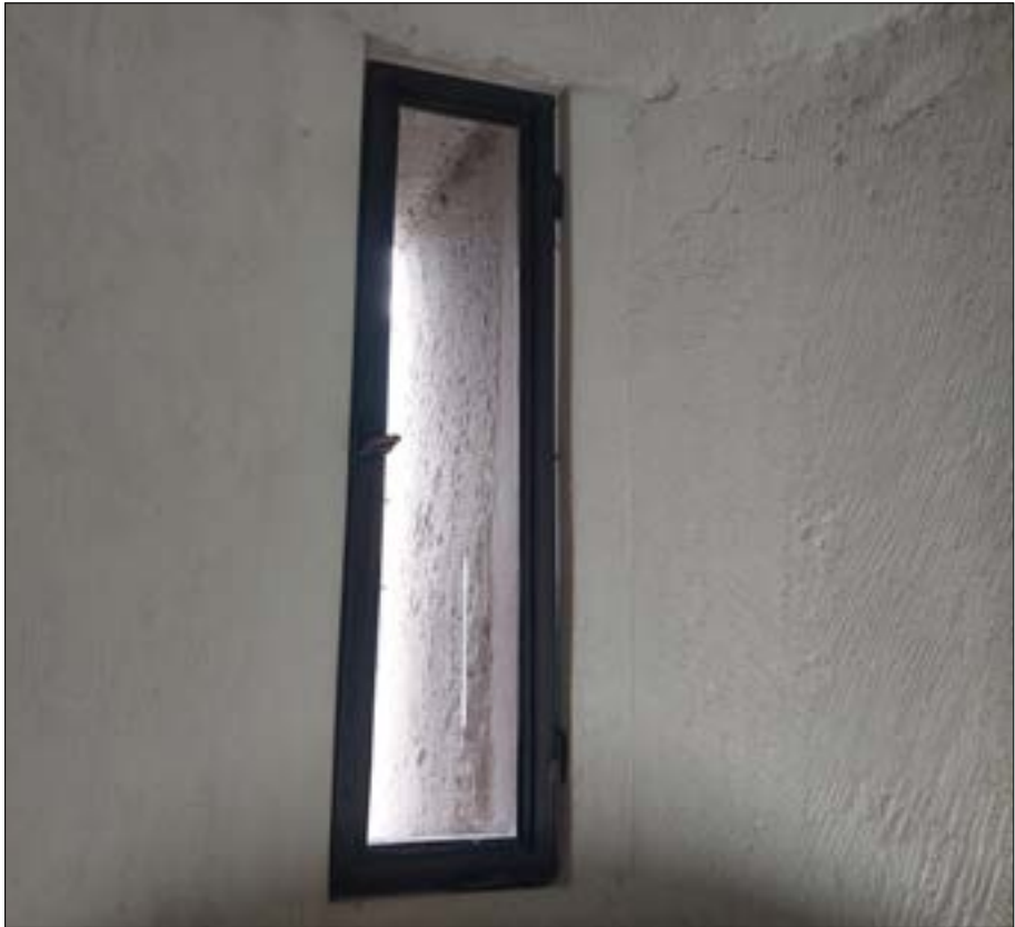
Fig. 51 Bronze casement window flush with stone wall, 2024
