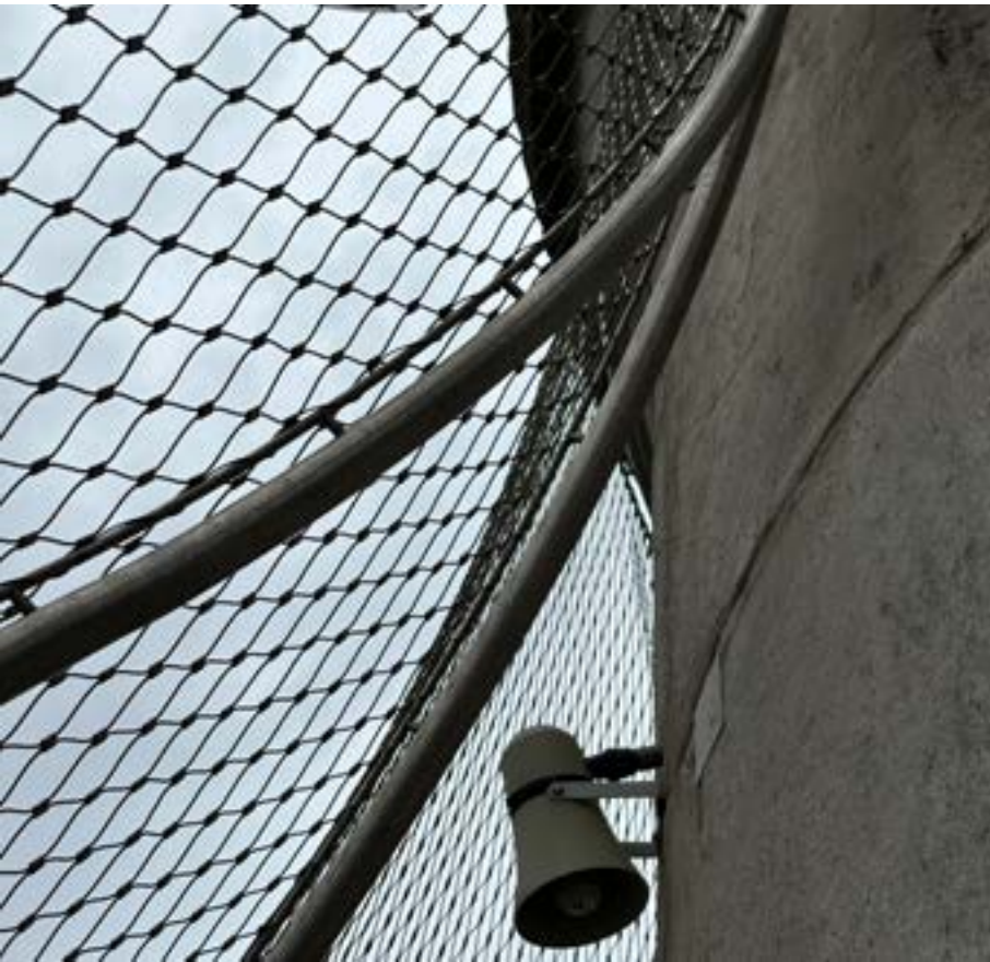
Fig. 91 Viewing platform speaker fixed to the stone Drum, 2024
