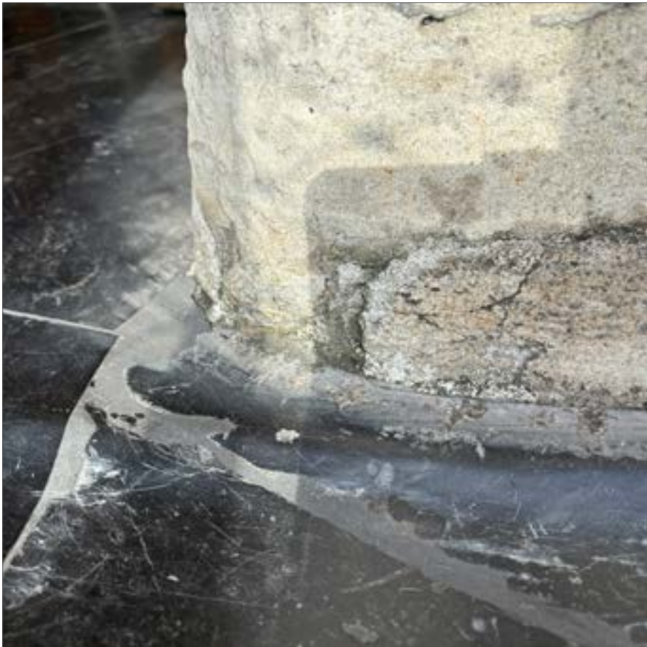
Fig. 9 & 10 Wide joint at the base of the Drum, 2024
