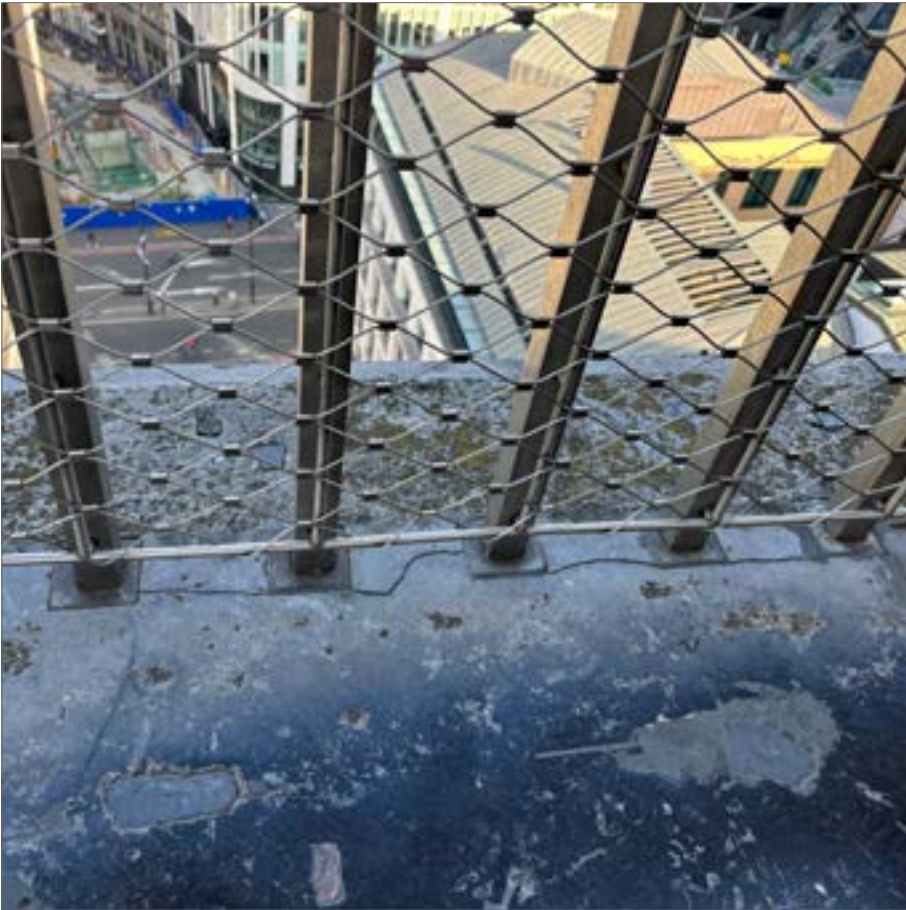
Fig. 12 Crack line along the base of balusters, 2024
