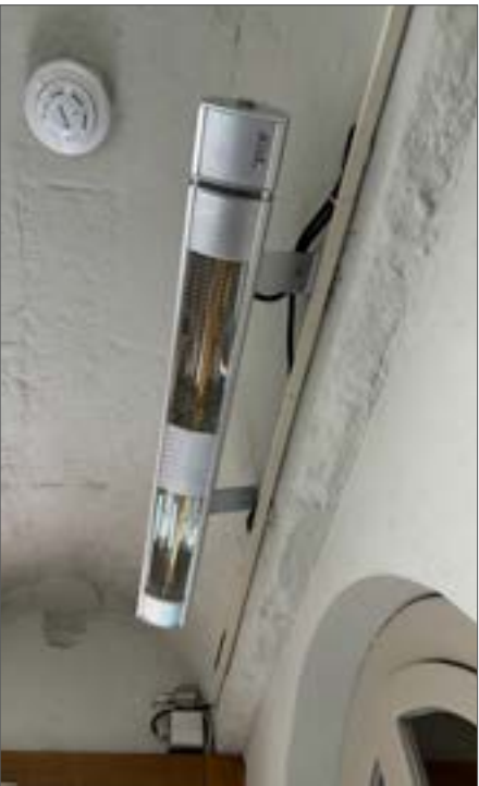
Fig. 84 Radiant electric heater, black cabling is visible, 2024
