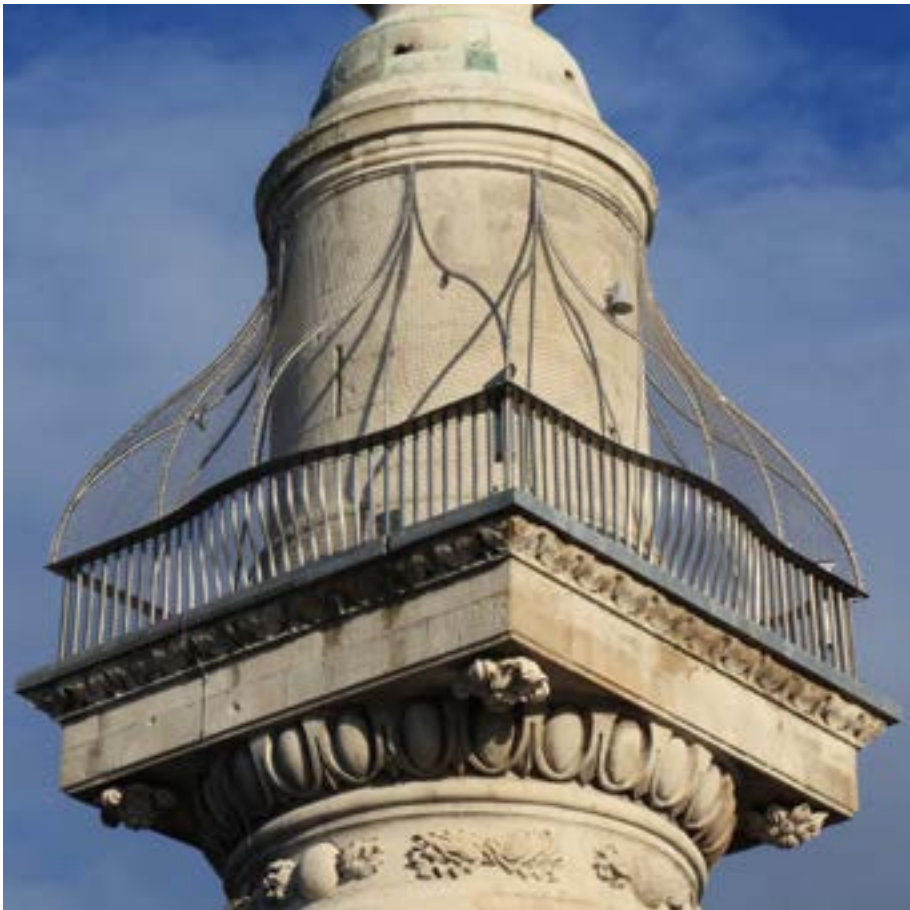
Fig. 78 Viewing platform stainless-steel cage & balustrade, 2009
