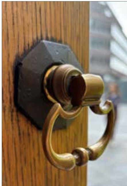
Fig. 26 Mortice interior escape latch, 2024
