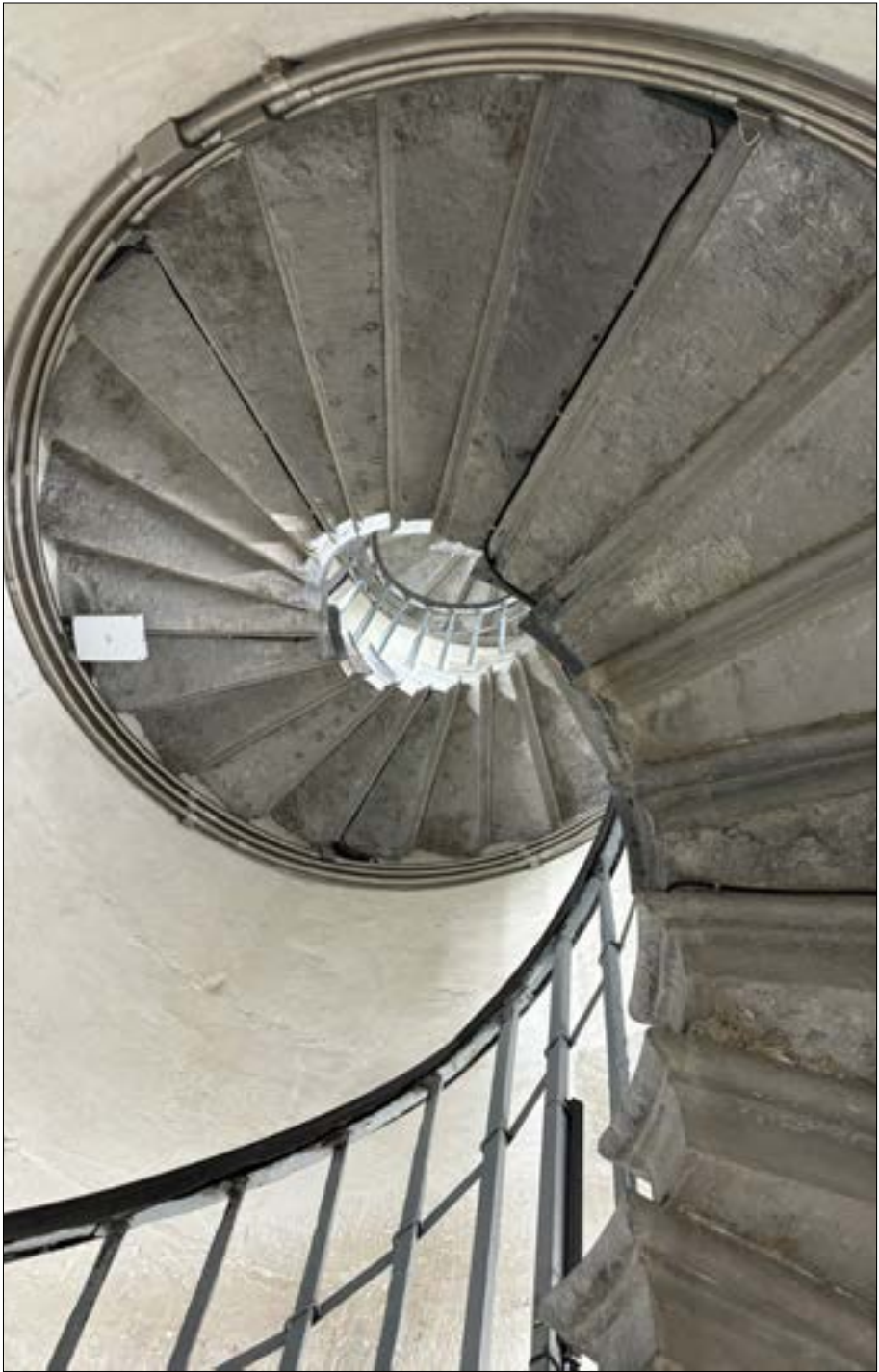
Fig. 60 Looking up at the underside of the stair treads at the original black limestone, 2024
