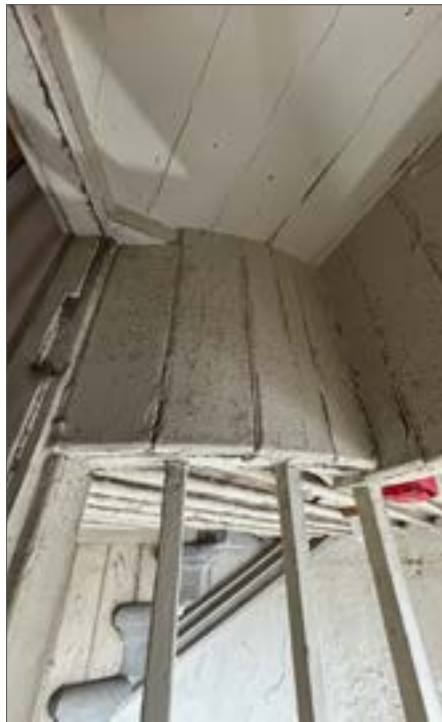
Fig. 51 Balusters lead-caulked into treads, 2024
