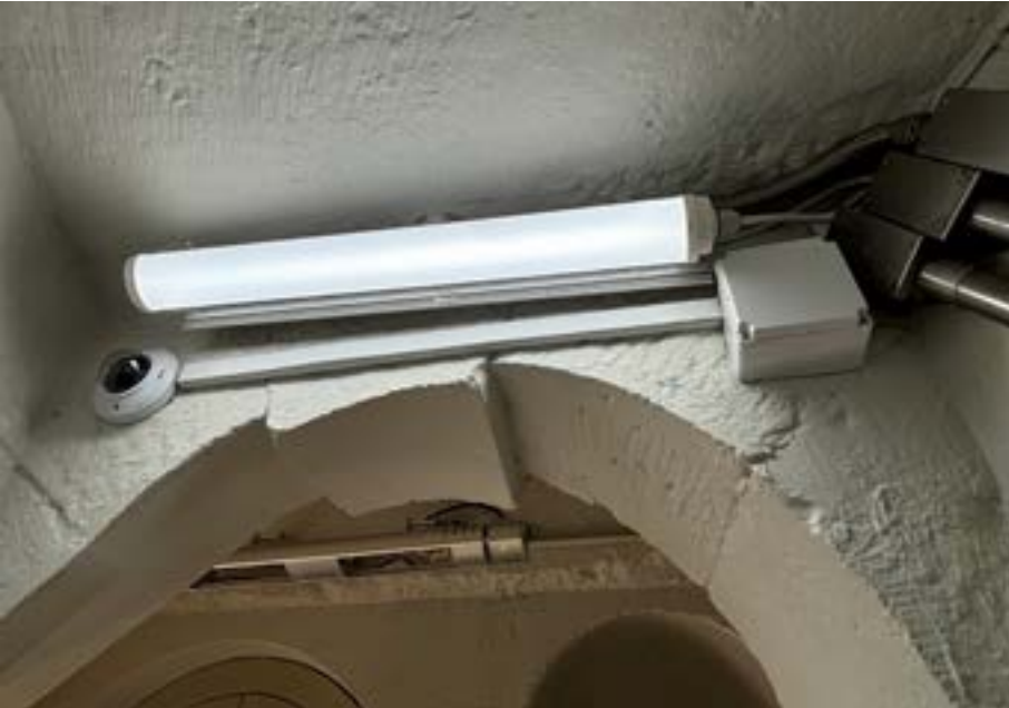
Fig. 98 Attendants recess strip light, CCTV plastic junction box & plastic conduit, 2024
