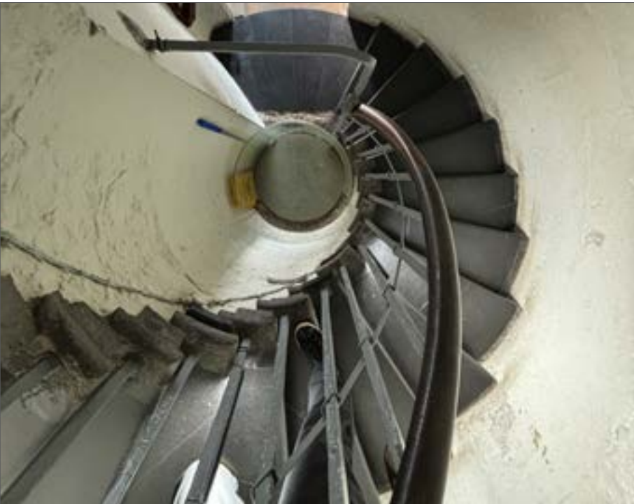
Fig. 71 Looking down the spiral staircase at the boarded-over oculus (circular floor opening), 2024
