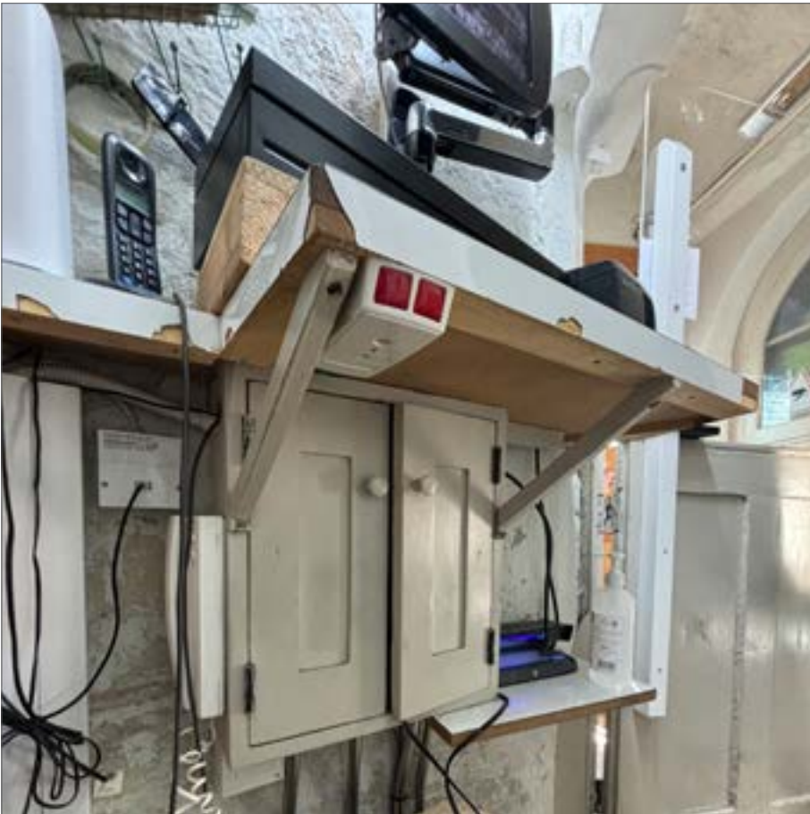
Fig. 65 The electrics' cupboard c.2009 can no longer contain all electrical services, 2024
