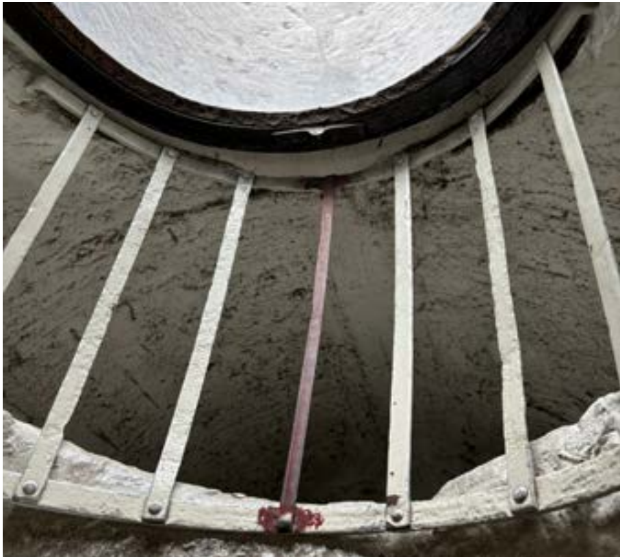
Fig. 83 Flat iron bars rivetted across a ventilation opening beneath the east oval window, 2024
