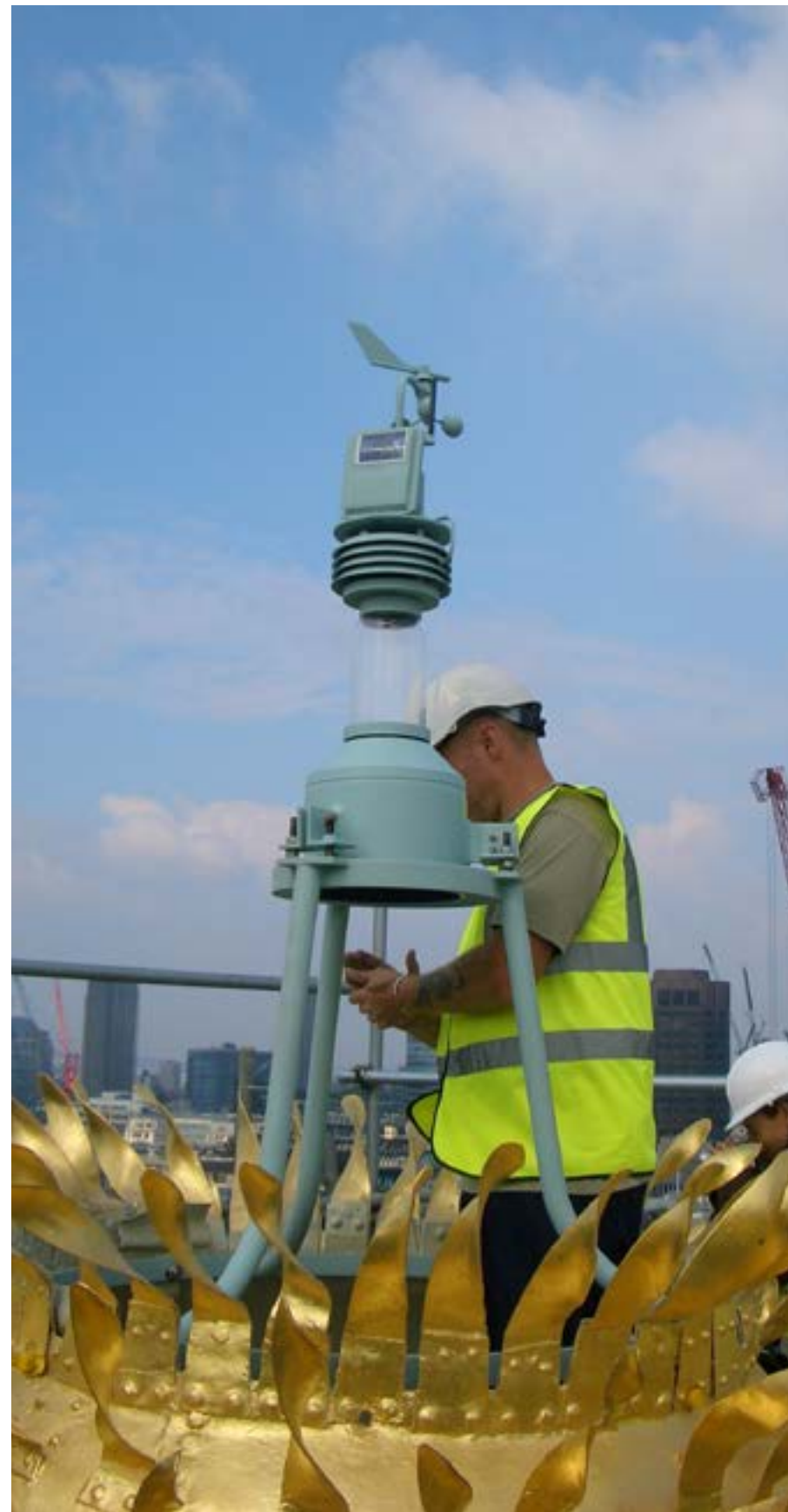
Fig. 112 Installation of the temporary camera, casing, weather station and steel support frame, 2008
