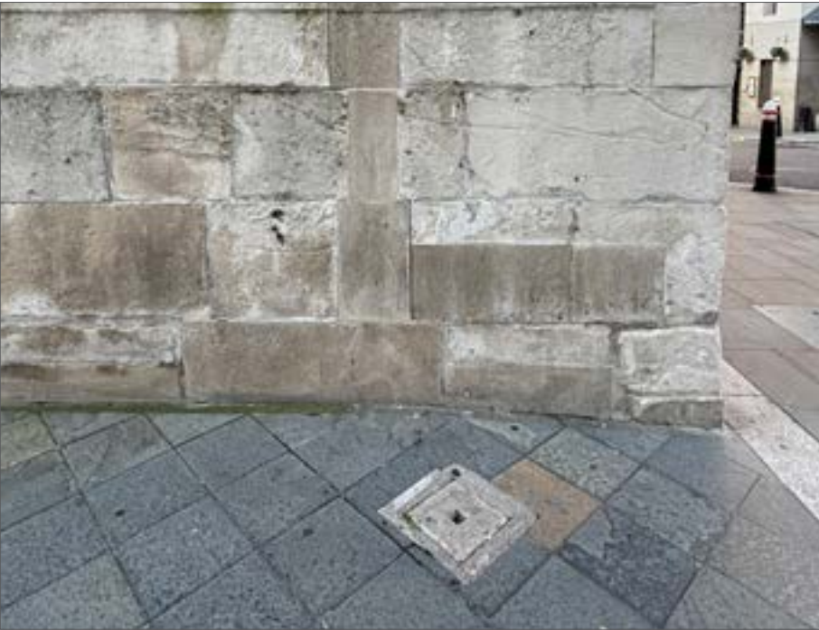
Fig. 108 North elevation down conductor, partly concealed, and test pit, 2024
