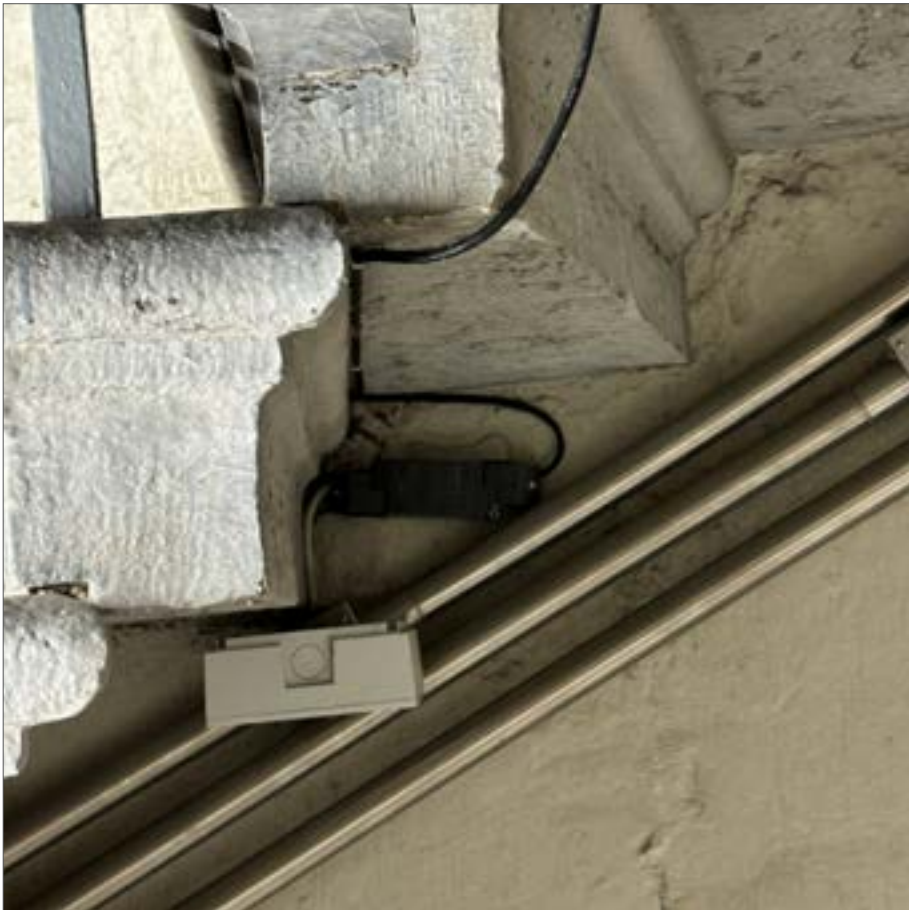
Fig. 99 Black cabling connecting a transformer to the replacement baluster lights, 2024
