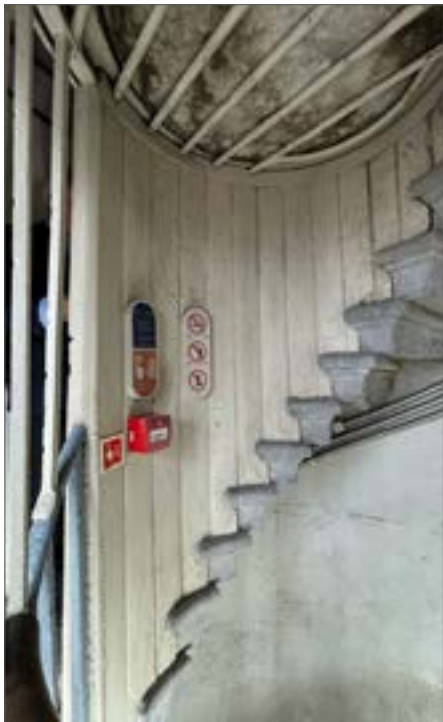
Fig. 50 Steel flat bends around baluster, 2024
