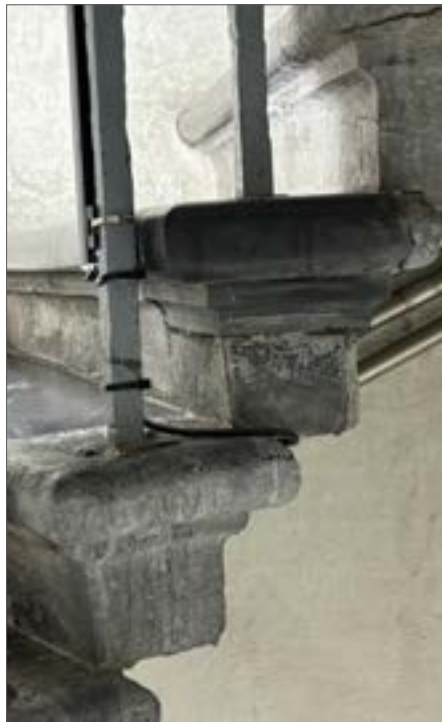
Fig. 41 Balusters lead-caulked into treads, 2024
