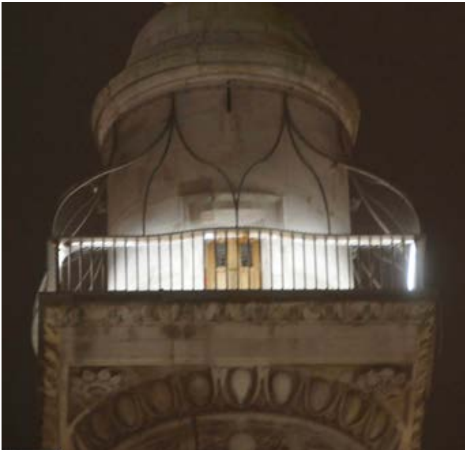
Fig. 93 LED lighting rope beneath viewing platform handrail, 2018
