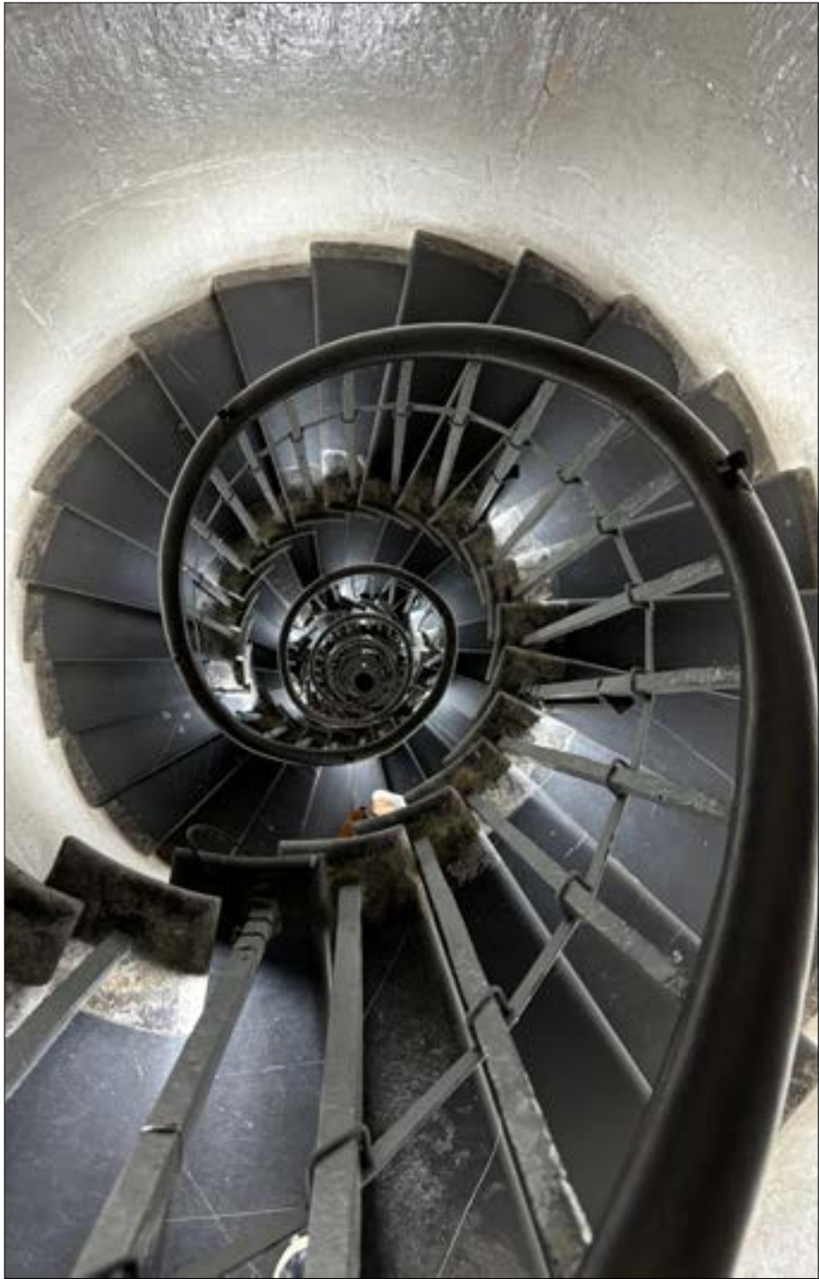
Fig. 59 Looking down the helical staircase showing stone insert repairs to all historic stair treads, 2024
