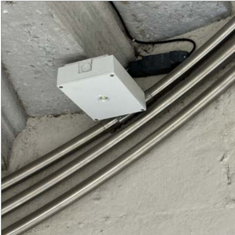
Fig. 100 Recent emergency lights in the stairwell, replacing baluster emergency lights, 2024
