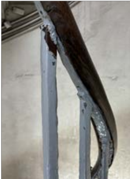
Fig. 43 Fixing of timber to ironwork, 2024
