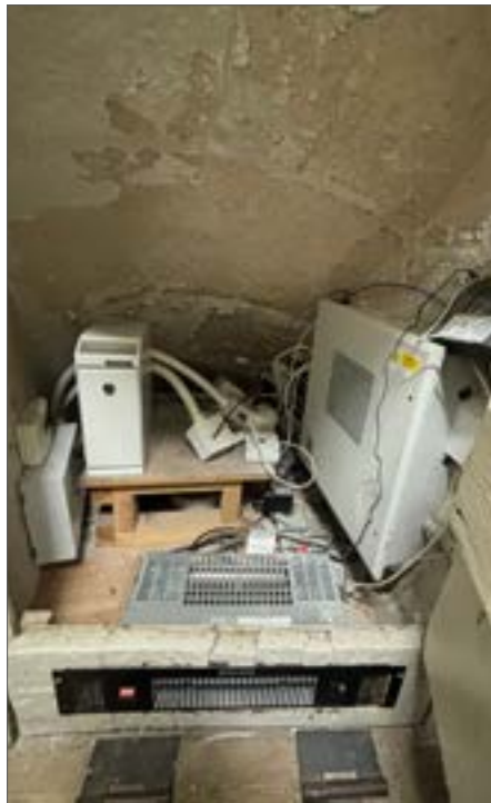
Fig. 87 Kick-space fan heater in skirting of cupboard, 2024
