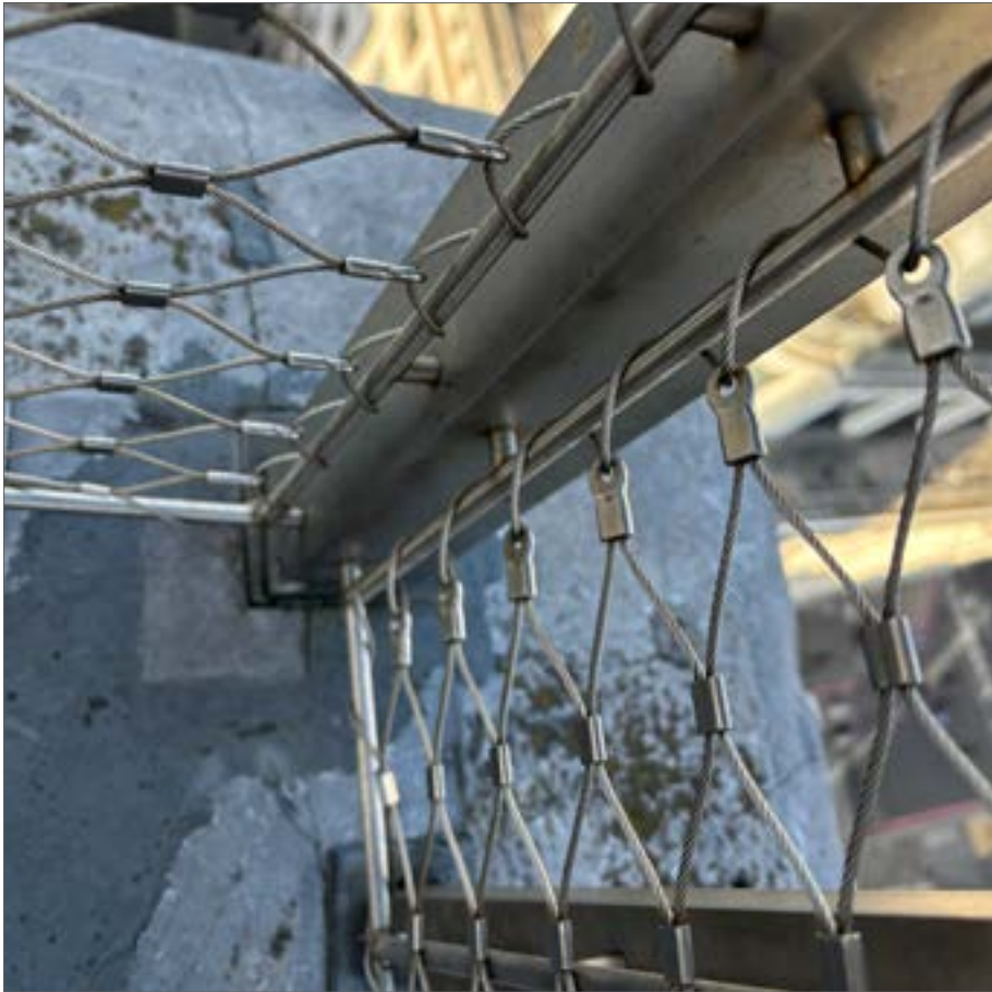
Fig. 13 Detail of a balustrade corner post, 2024
