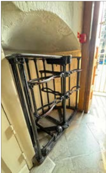
Fig. 69 Turnstile in north recess (arms missing), 2024
