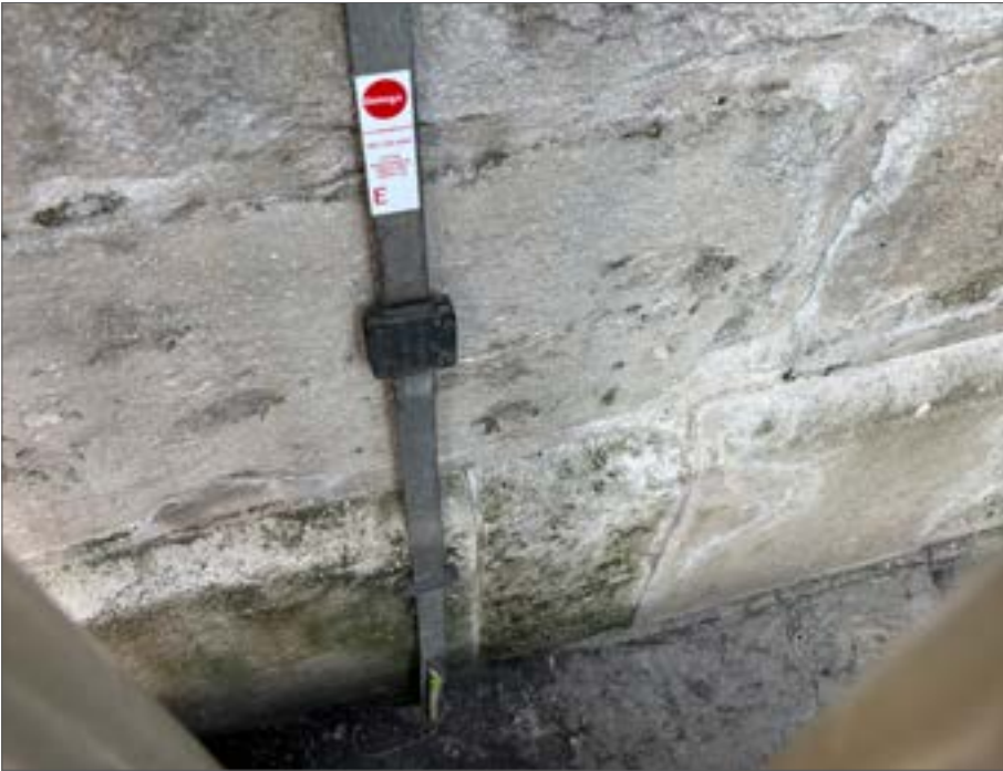
Fig. 109 East elevation down conductor, surface mounted, 2024
