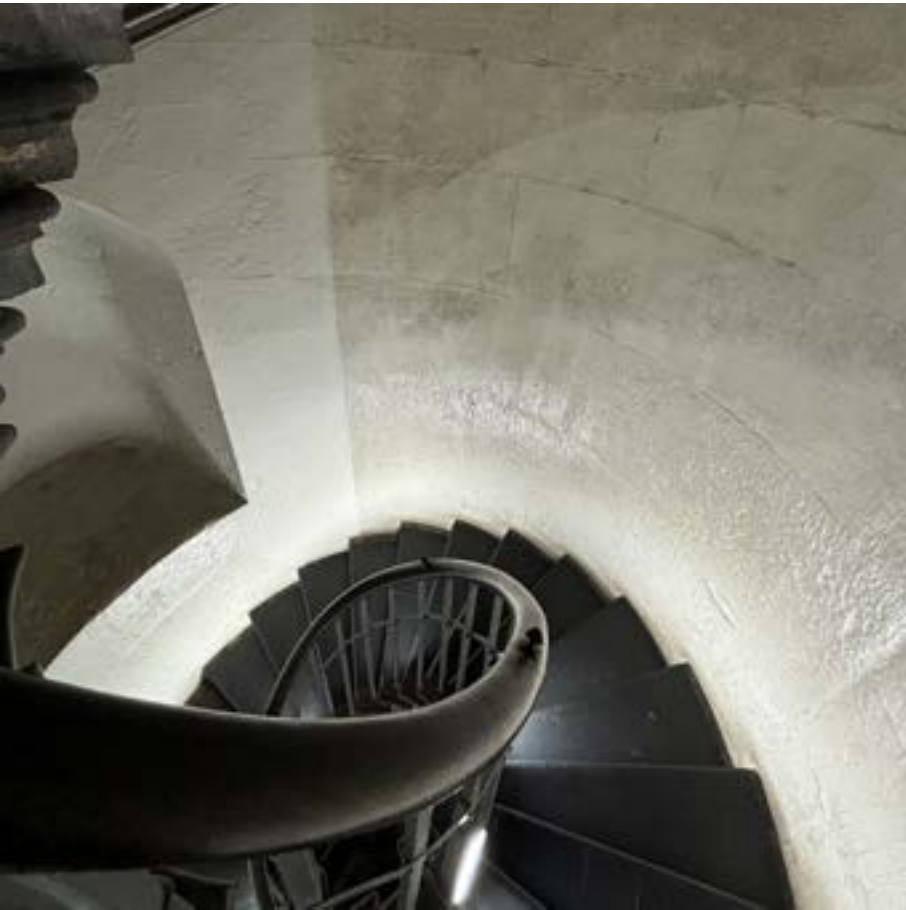
Fig. 85 Staircase balustrade curved oak handrail, 2024
