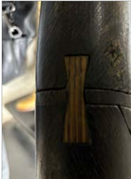
Fig. 46 Recent unstained butterfly joint, 2024
