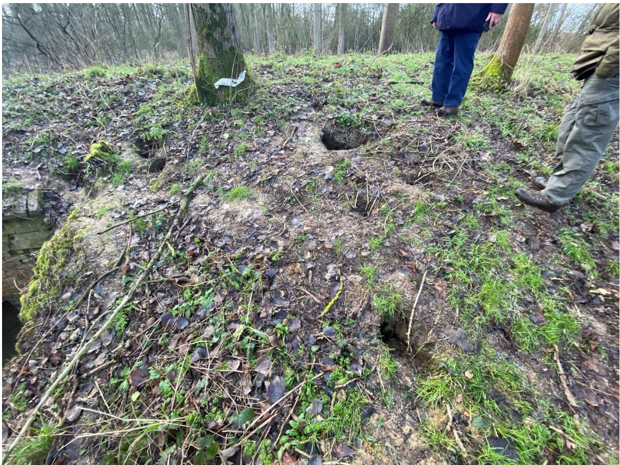
Plate 2 Example of damage to the dam from protected species, near to one of the culverts.
