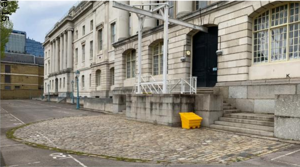
Image 1: Existing Central Steps
