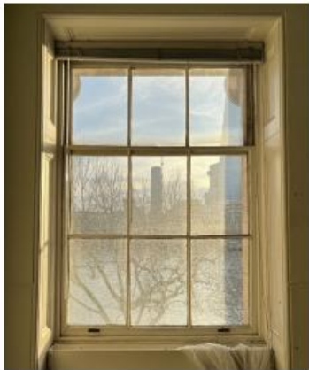
WWI.07 3/6 sash, deep timber panelled reveal
