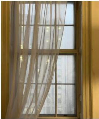
WCI.60 6/6 sash, slim timber panelled reveal
