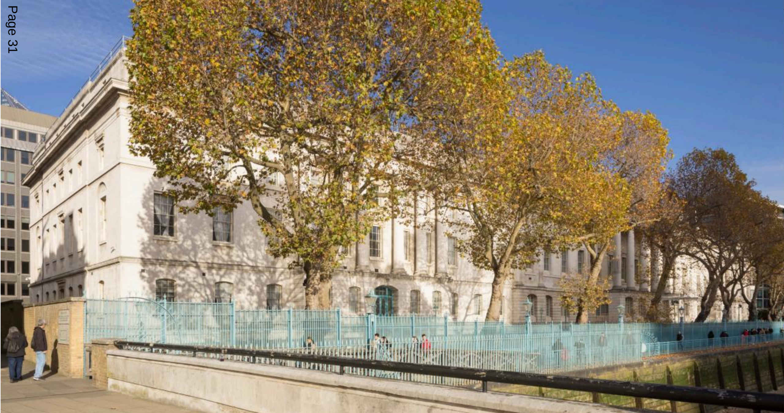
Existing CGI view from Billingsgate Walk
