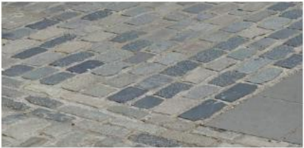
Adaptively re-used granite setts
