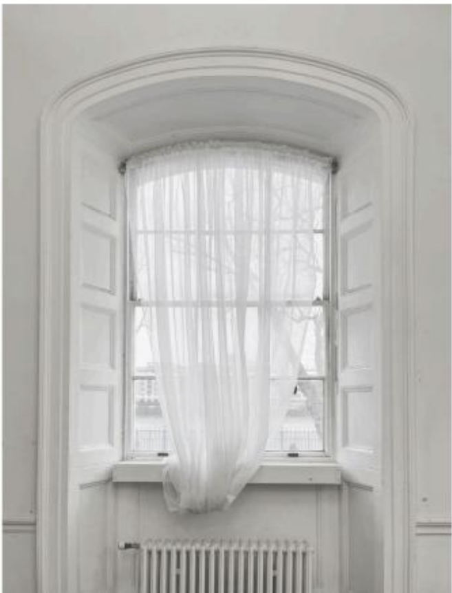
Image 1: Existing Window and Bomb Blast Curtains
