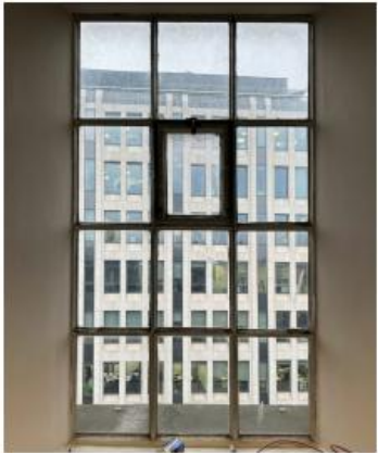
WCT.59 12 casement window, 1 no. openable panel
