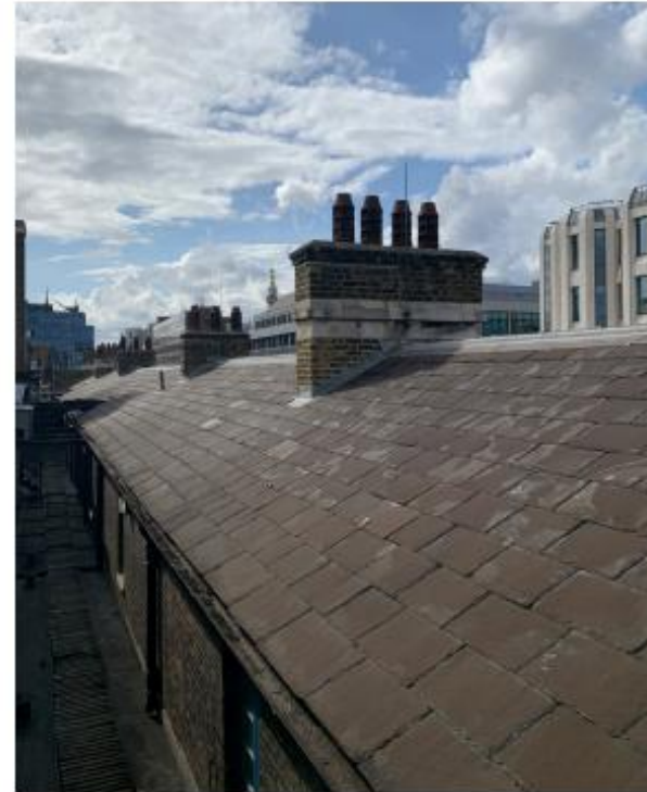
Image 2: Existing Rear Slate Roof
