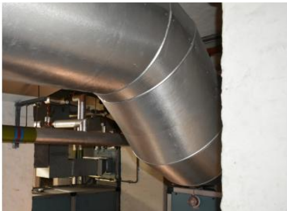
Image 4: Existing Ductwork
