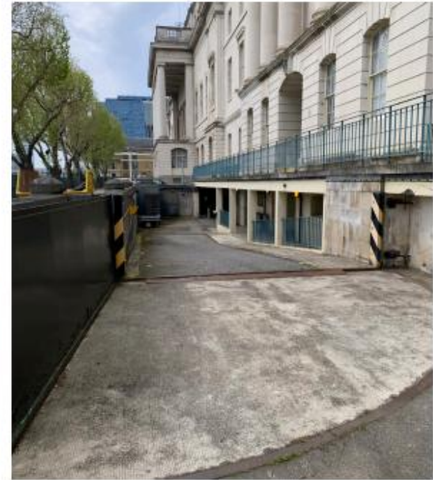
Image 3: Existing Ramp to Basement
