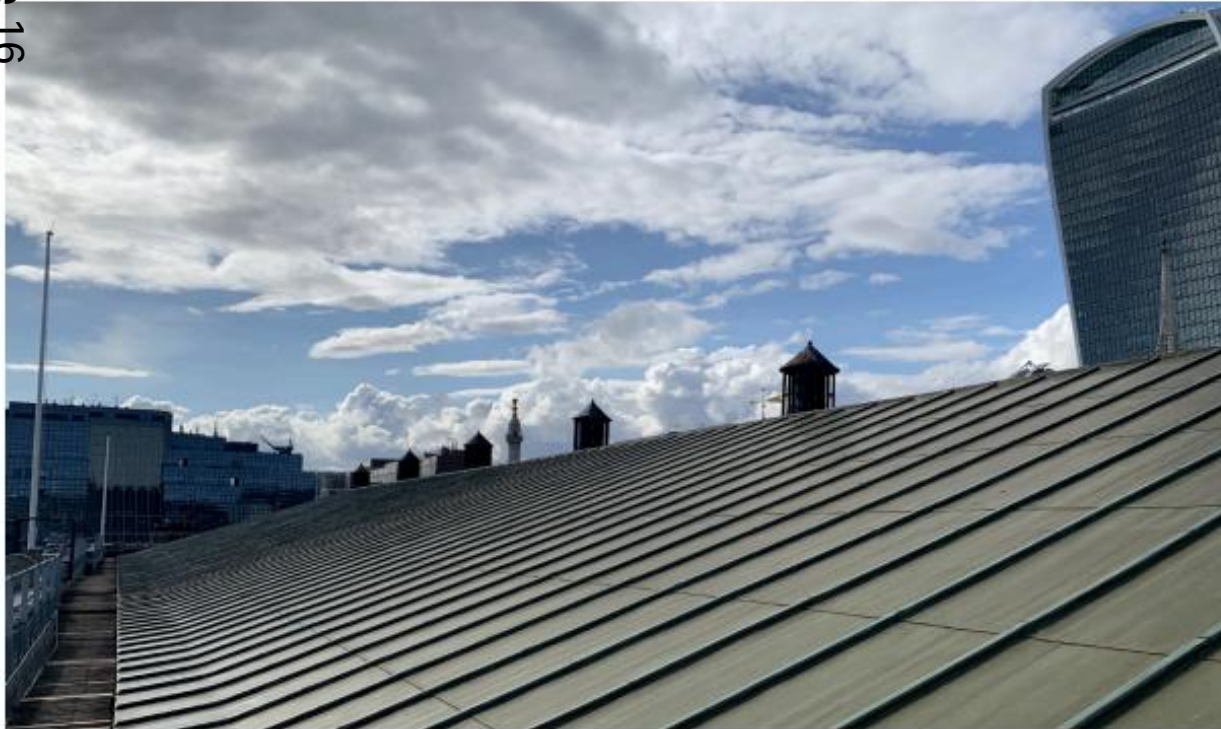
Image 1: Existing Central Copper Roof
