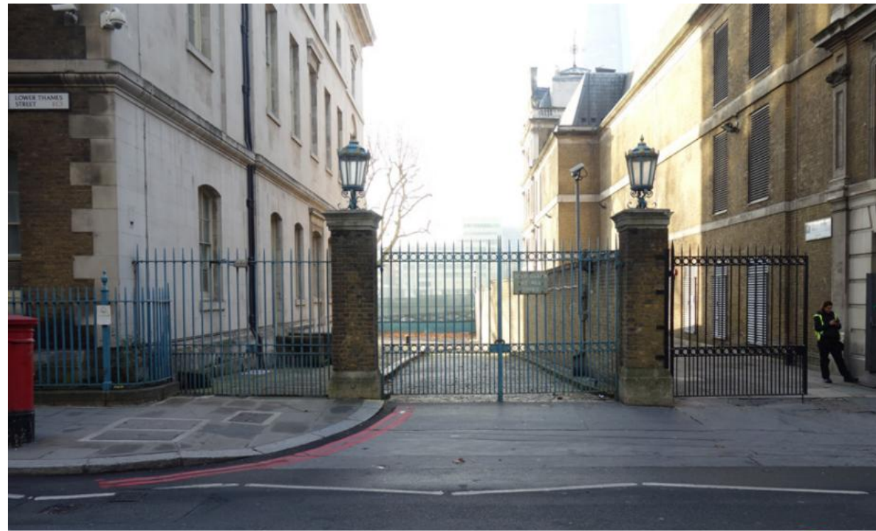
Image 2: Existing West Entrance
