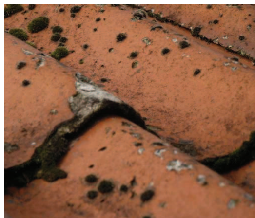
Friable roof surface (4.14)
