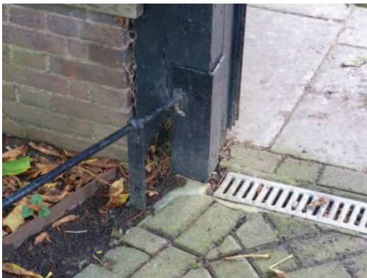
Rotten oak post adjacent to drainage channels (2.20). Steel reinforcement bolted to brickwork(2.21)
