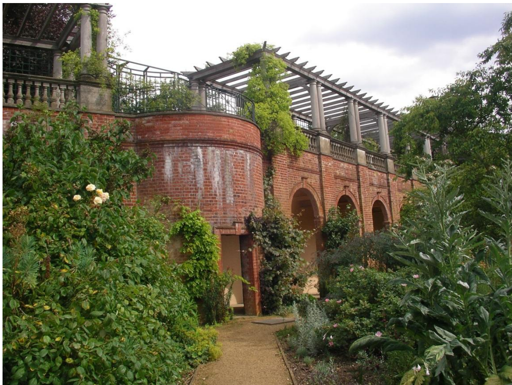
Section 1: The rotunda feature showing unsightly efflorescence.
