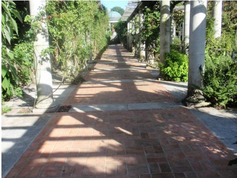
Section 2: showing renewed brick pavements and planting beds set into the structure.
