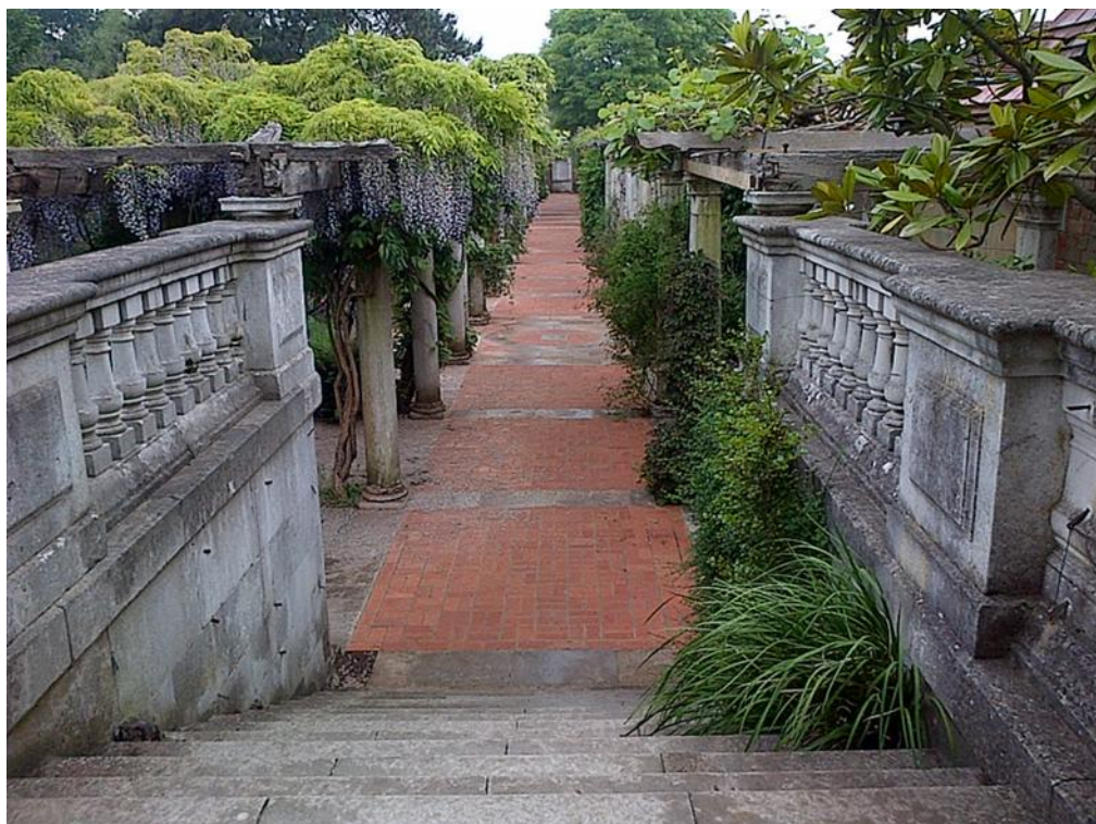
Section 2: general view showing renewed brick pavements.
