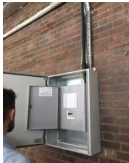
Engineers inspecting the newly installed cabinets implemented as part of cabling upgrade works
