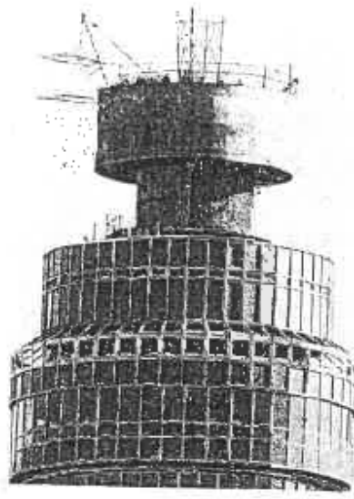
Raising a section of the steel tower by derrick pole at the top of London's Post Office tower.
