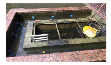
Intake pipe by The Postern – rediscovered and uncapped, after much sludge removal (almost 6ft deep)
