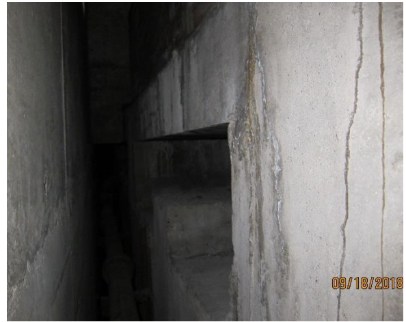
Interface of Defoe House structure with LUL running tunnel, showing a clear gap of \sim 400\text{mm}
