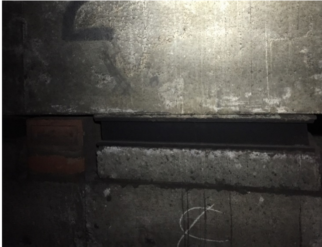
Figure 13 – Resilient Rubber Bearings within the Concrete Structure
