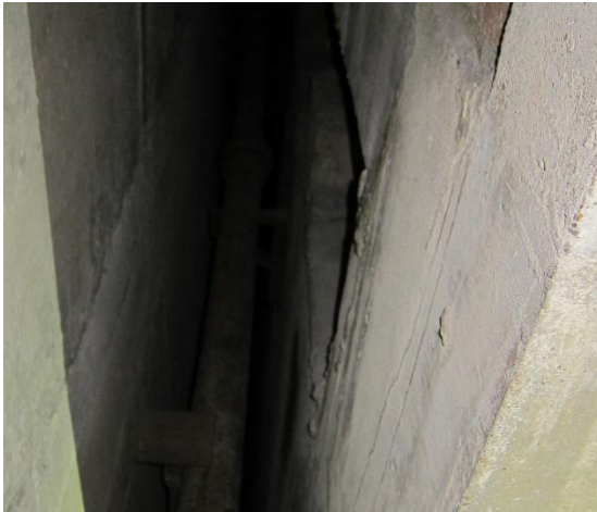
Interface of Defoe House structure with LUL running tunnel, showing a clear gap of \sim 400\text{mm}
