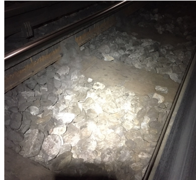
Figure 2 – Bullhead Rail on Timber Sleepers
