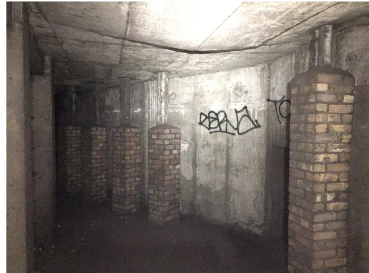
Figure 16 – Supporting Brick Columns
