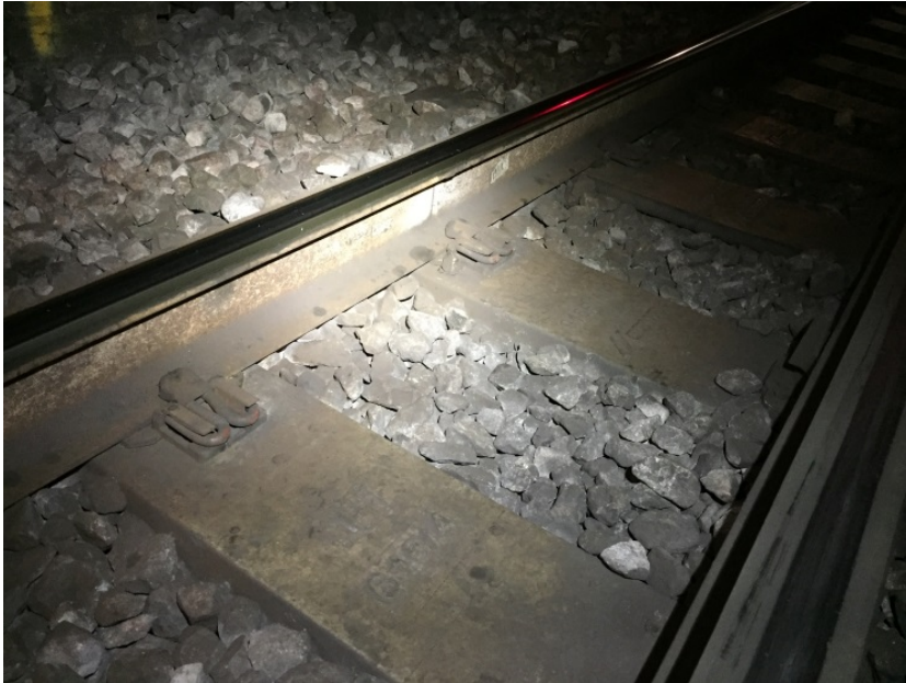
Figure 1 – Flat-Bottom Rail on Concrete Sleepers
