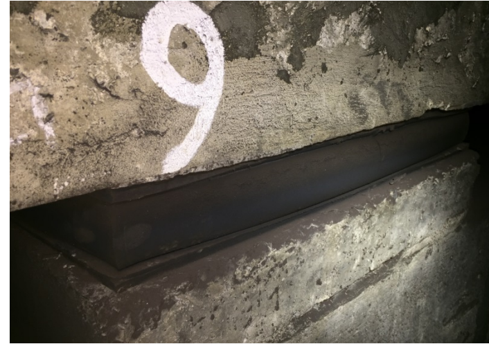
Figure 14 – Resilient Rubber Bearings within the Concrete Structure
