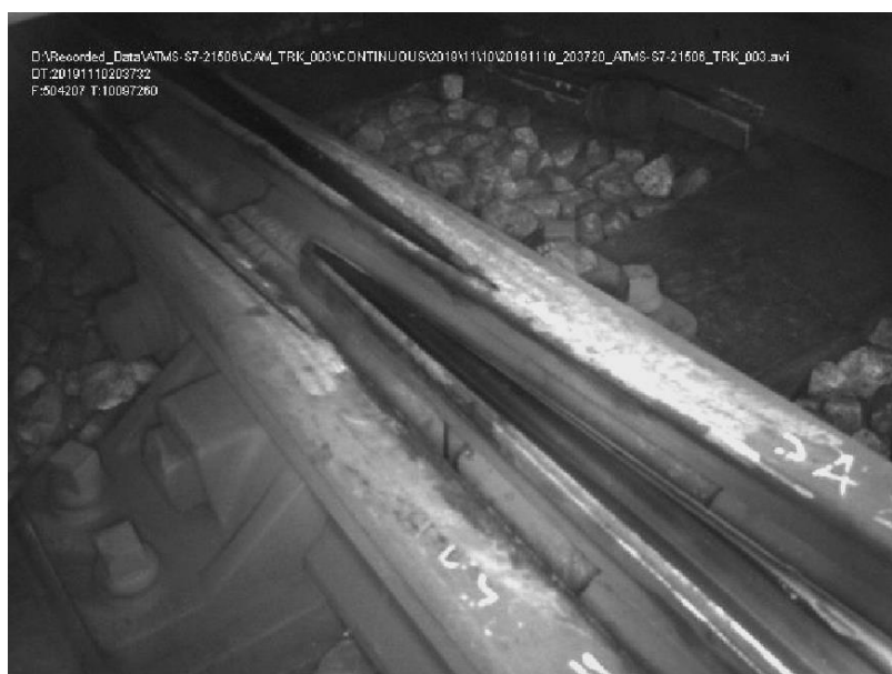
Figure 2 – Rail discontinuity (nose of points 35A) on the right hand rail at LCS M134/MORLO 466m
