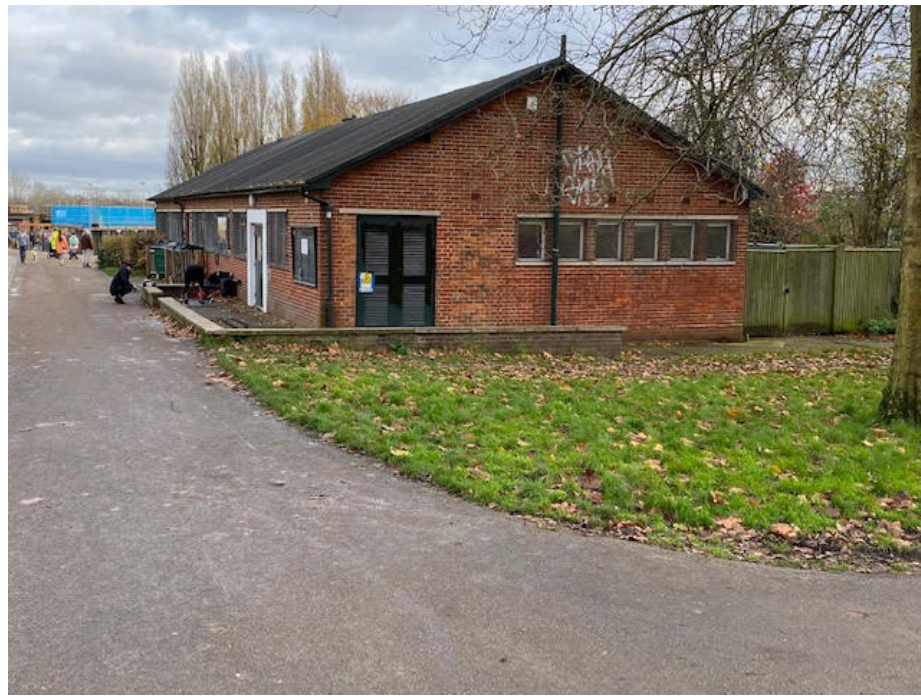
Hive Building - Change white paint on all windows and main door surround to mushroom.
