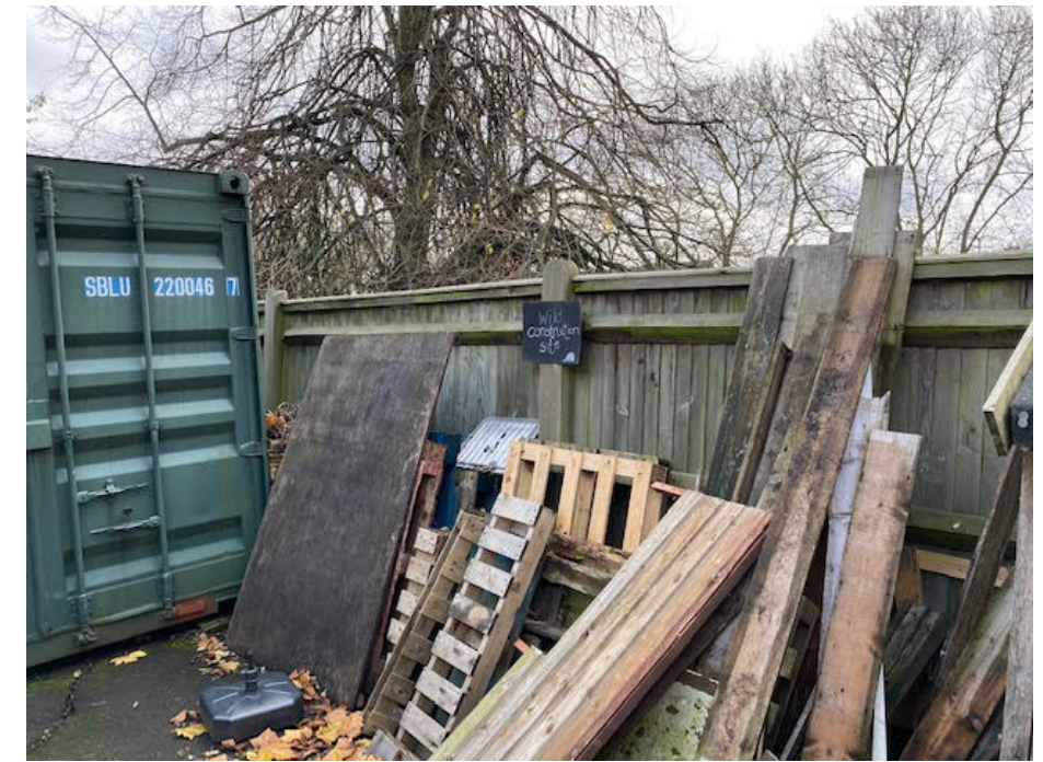
Realign external enclosure fence and move approx 2m further from building. Change fence to horizontal featherboards with top 300mm as mesh or lattice pattern.
