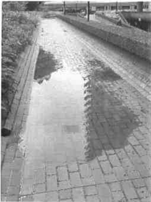
Flooding on the new Beech Gardens Highwalk
