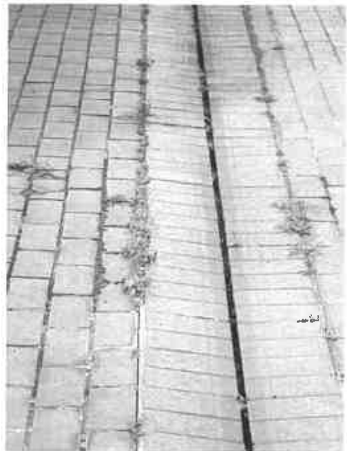
Plants in mortar joints on Cromwell Highwalk
