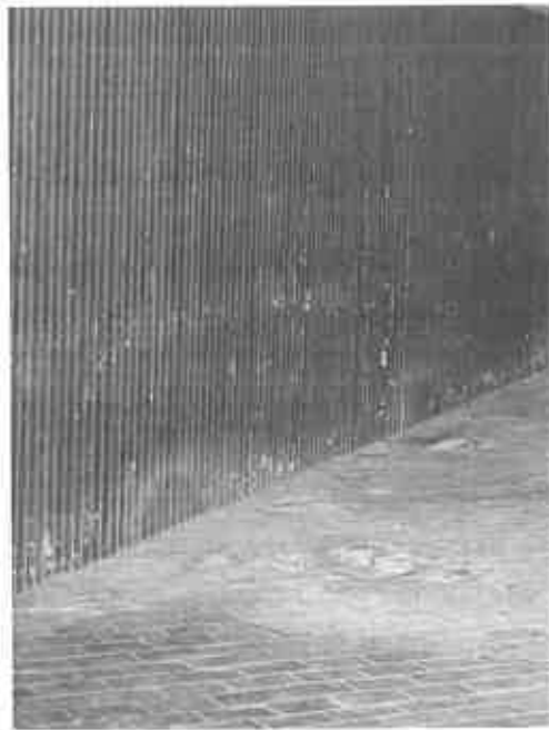
Railings unpainted for at least 20 years and 20 mm thick calcination on Defoe Place
