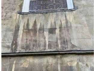
Figures 21 & 22. Details of cracking to the render and previous repairs on the west elevation of the Great Hall.
