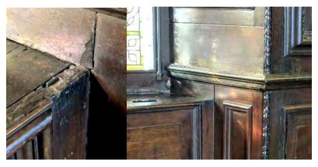
Figure 13: Missing internal sill boxing beneath the Cranmer window. Trimmed panel rail with section through mortice/tenon clearly visible.
