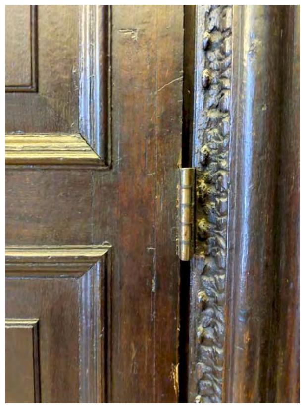
Figure 15: H-L (or H-Hinge) shadow still visible to the bi-folding doors. Later strip applied to edge to modify size.
