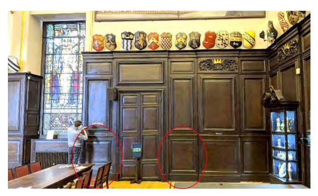
**Figure 12**: **Panelling to the north-west of Stationers' Hall.** The panel to the RHS of the Cranmer window affords transition between the two panelling types, higher skirting to the south off the hall achieved through a reduced lower panel (highlighted)
