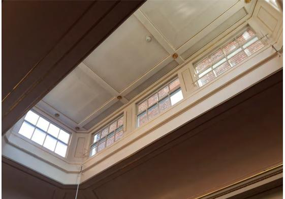
Figure 9: Glazed Lantern seen from inside the Card Room.
