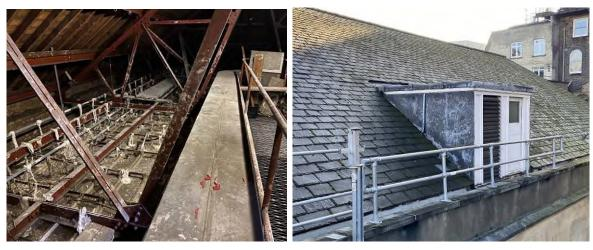
Figures 50 & 51. Details of the ducting in the roof and the large external louvred vent.
