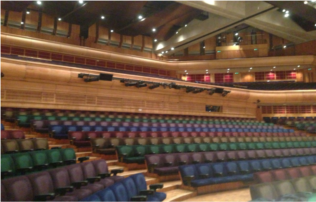
Auditorium 2017, showing new panelling and convex timber fascias on gallery fronts.
