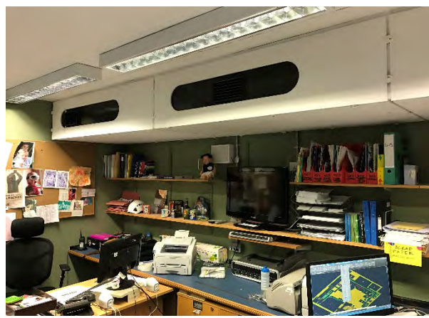
Original oval slotted duct detail
