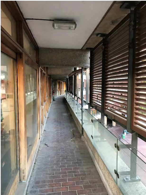
Original external façade windows and screens remain, with exposed uncoated concrete elements.
