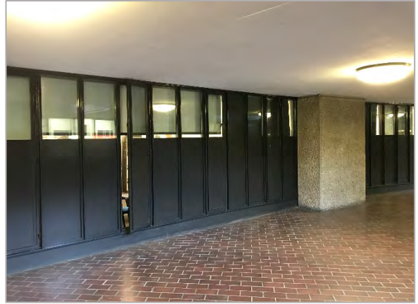
Offices surrounding Frobisher Crescent walkway, showing original close mullioned façade screen
