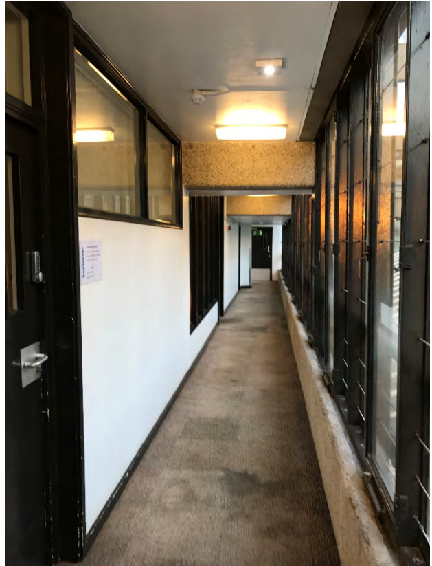
Original external façade windows and screens remain, with exposed uncoated concrete elements.
