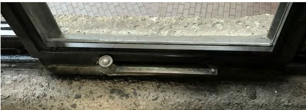
Window detail with new double glazing
