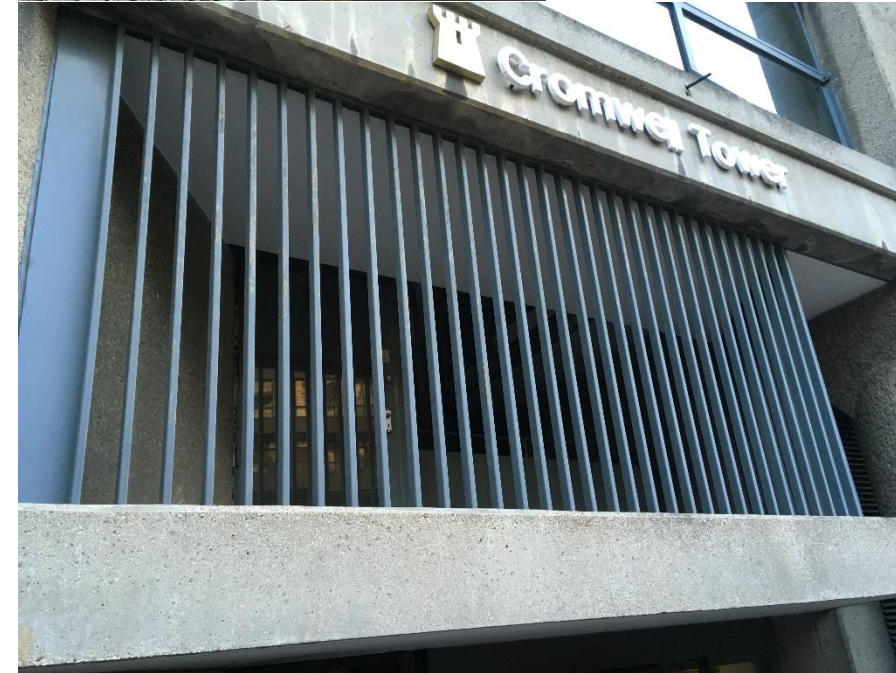
Figure 25: Permanent opening at the bottom of the firefighting stair at Podium Level
