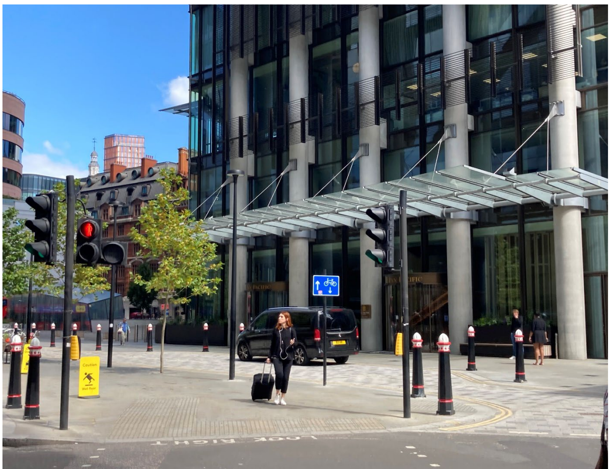
After: The raised carriageway in granite setts on Houndsditch.
