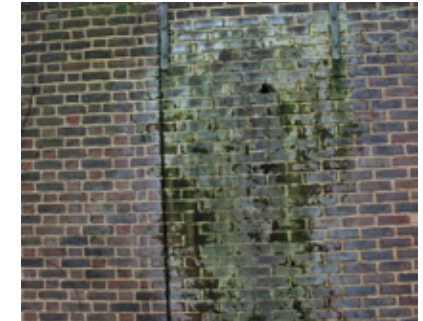
Staining on the brickwork of the maintenance area
