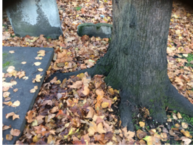
Root spread causing damage to tomb
