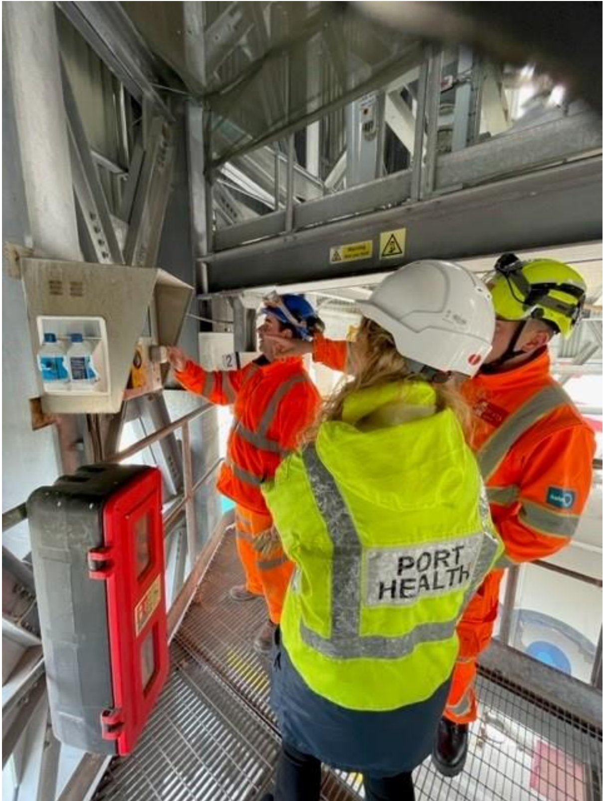
Photograph 4: Checking operation systems at Sheerness
