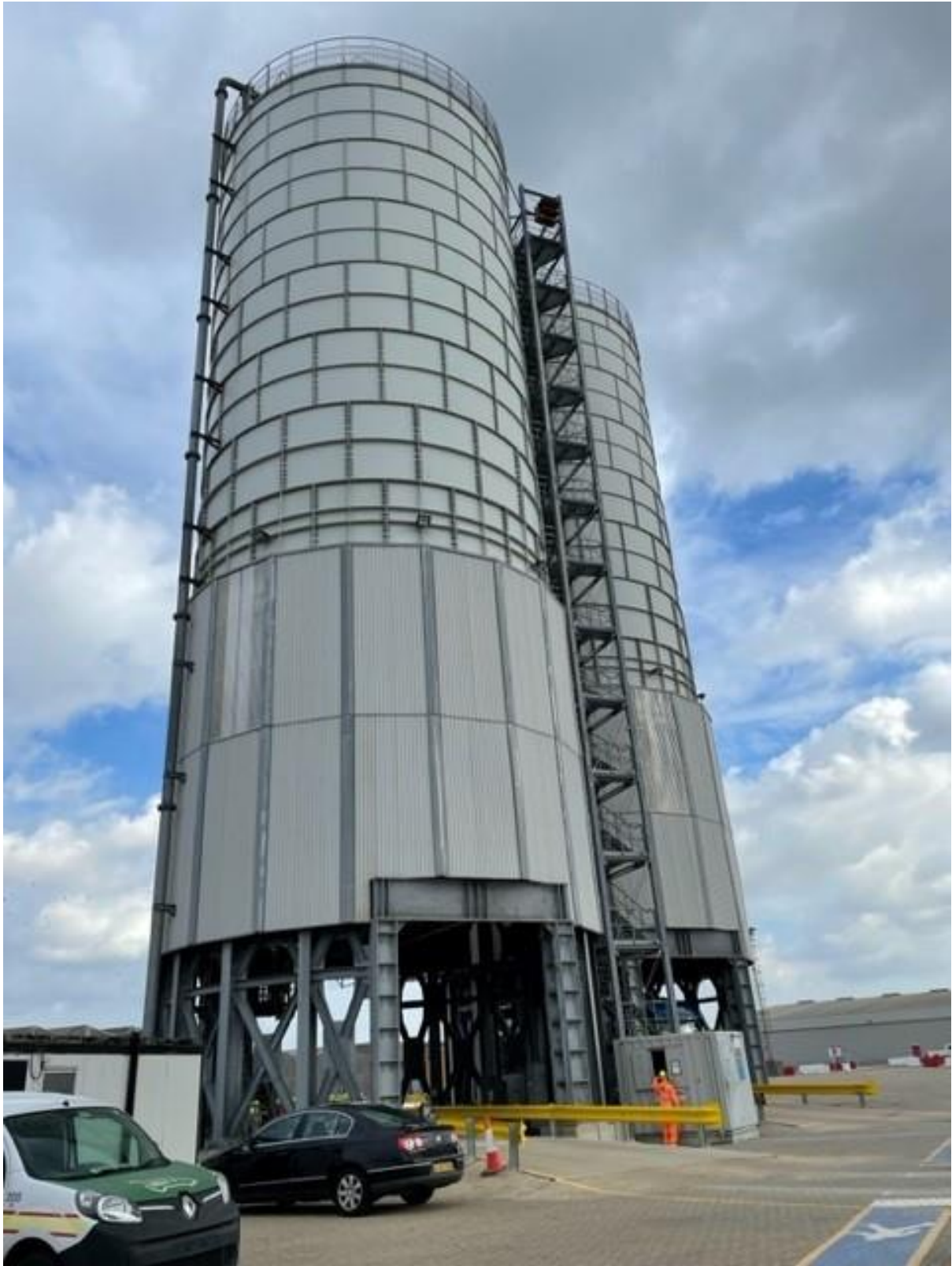
Photograph 3 : Silos at Sheerness
