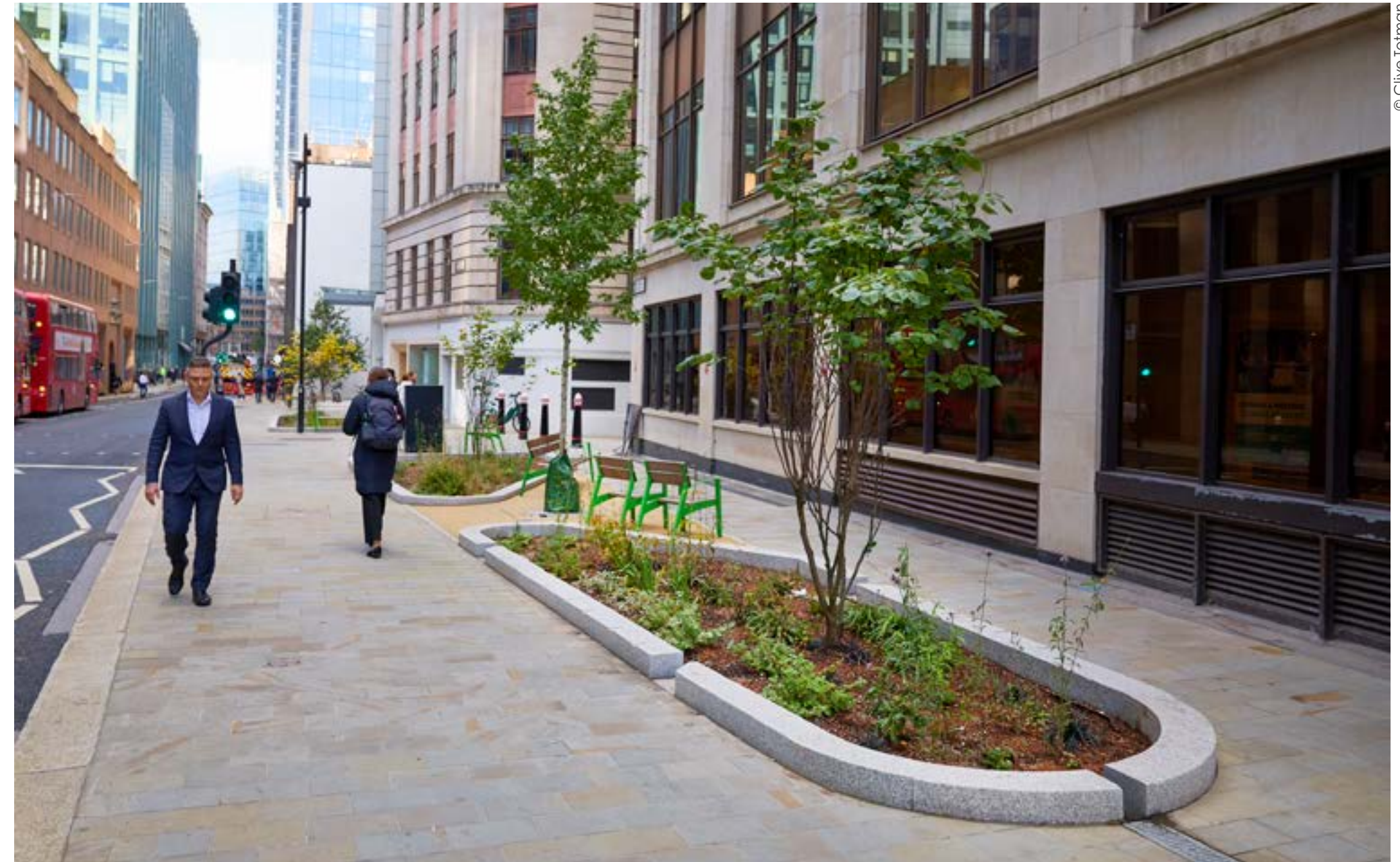
Bevis Marks SuDS: Future proofing our streets to flooding. Rain gardens in the east of the City capture and store surface water, interconnected with permeable paving and featuring ZINCO, a medium used for its lightweight and hydraulic efficiencies.
