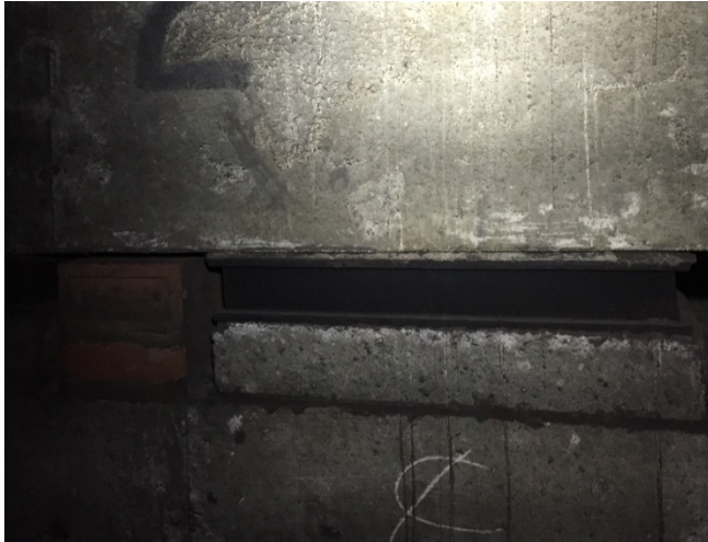
Figure 13 – Resilient Rubber Bearings within the Concrete Structure
