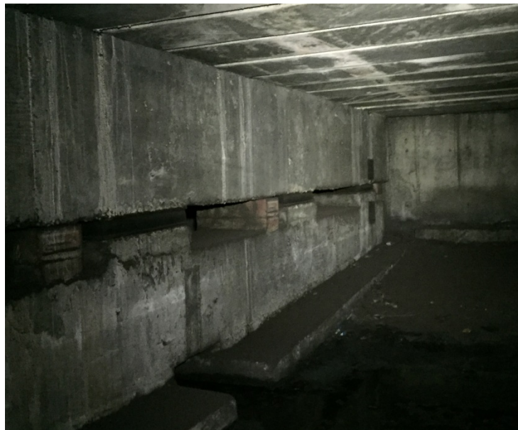
Figure 11 – Concrete Structure Supporting the Track
