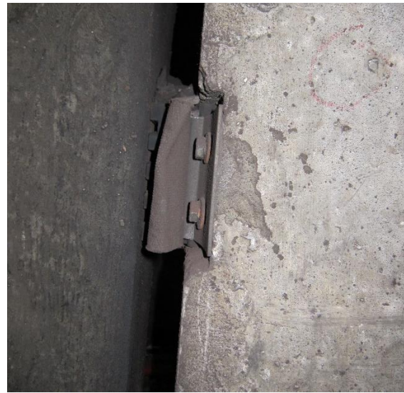
Flexible connection at 'pinch point'
