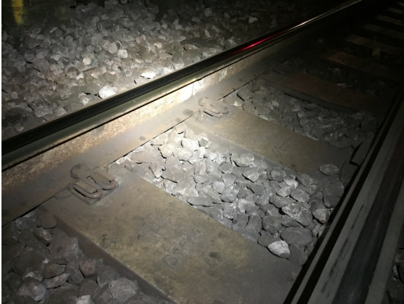
Figure 1 – Flat-Bottom Rail on Concrete Sleepers
