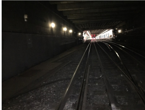
Figure 7 – Metal Grills on Concrete Running Parallel with Rails
