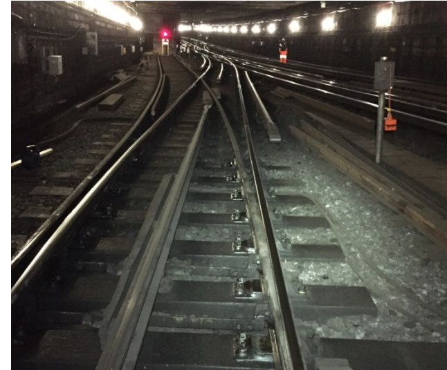
Figure 4 – Sidings Flat-bottom Rail on Concrete Sleepers from Platform 3
