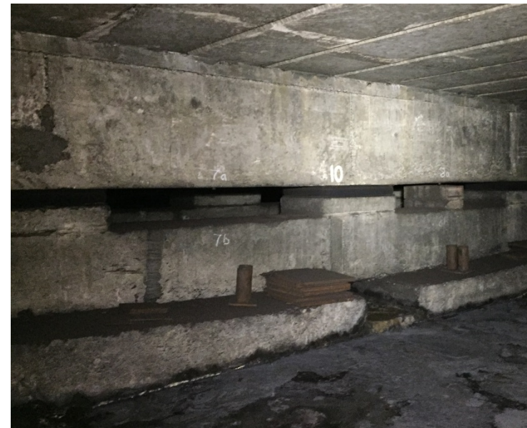
Figure 12– Concrete Structure Supporting the Track
