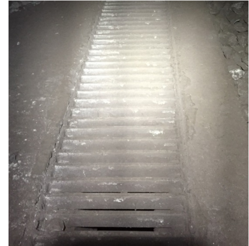
Figure 8– Metal Grills on Concrete Running Parallel with Rails
