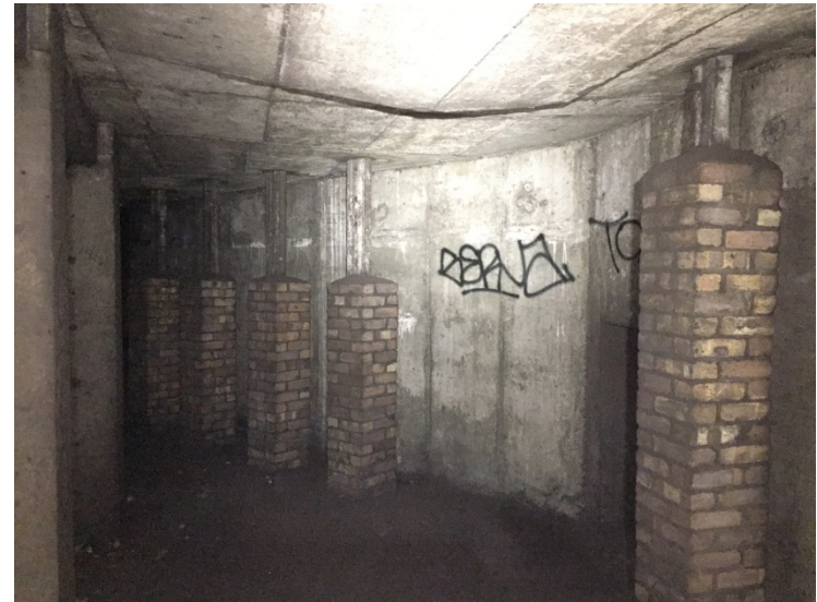
Figure 16 – Supporting Brick Columns
