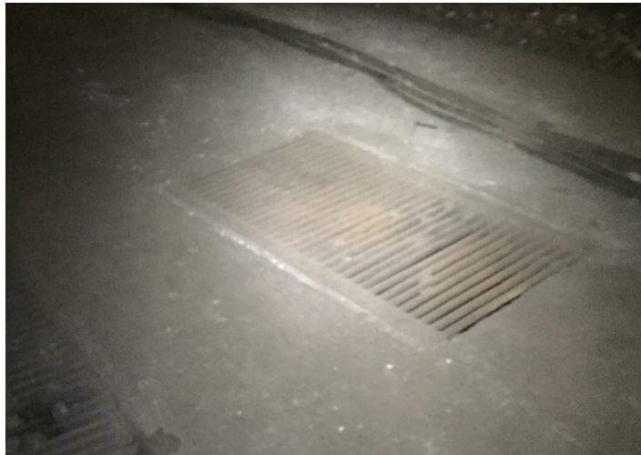
Figure 9 – Removable Grills to Access Chamber
