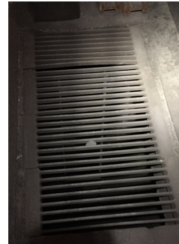
Figure 10 – Removable Grills to Access Chamber
