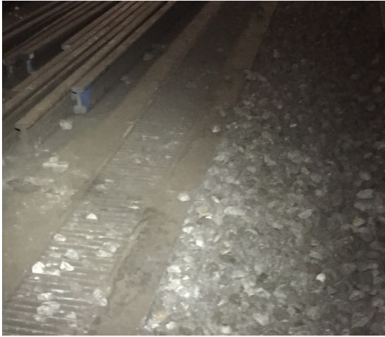
Figure 6 – Metal Grills on Concrete Running Parallel with Rails
