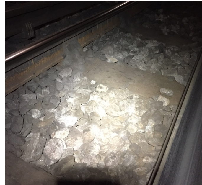
Figure 2 – Bullhead Rail on Timber Sleepers
