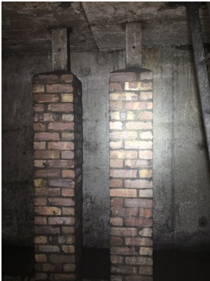
Figure 15 – Supporting Brick Columns
