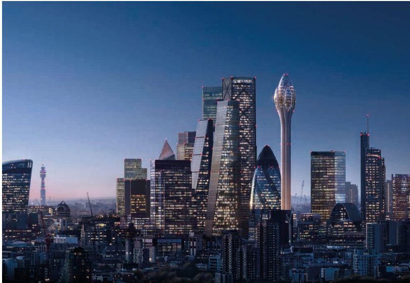
Figure 11 – Image illustrating the proposed lighting strategy for The Tulip with three layers of light including ‘Interior glow’, lighting of the linear elements and ‘Base uplight’
