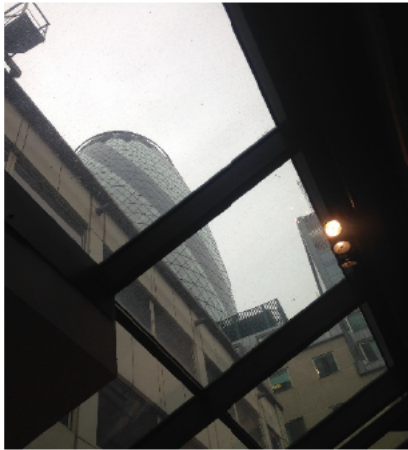
Figure 9 - View of 30 St Mary Axe through the glass roof of the Synagogue Annexe facing west
