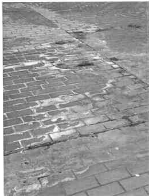
Paving on the Sculpture Court
