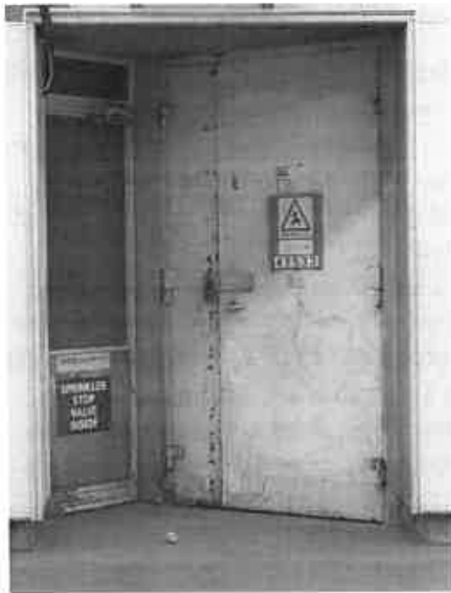
Door to the Estate from Beech street
