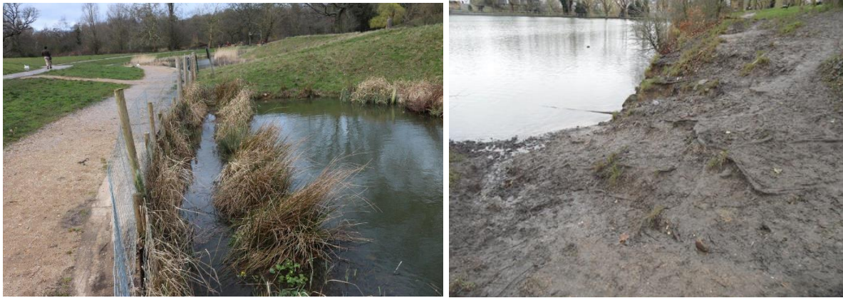
Figure 3: Boating pond plant damage and Hampstead No.2 dog erosion.
