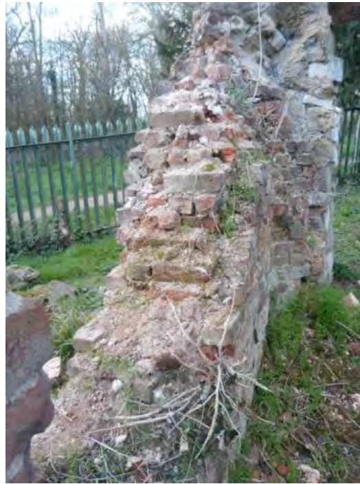
Fig 4: loose bricks on west side of opening of Zone A
