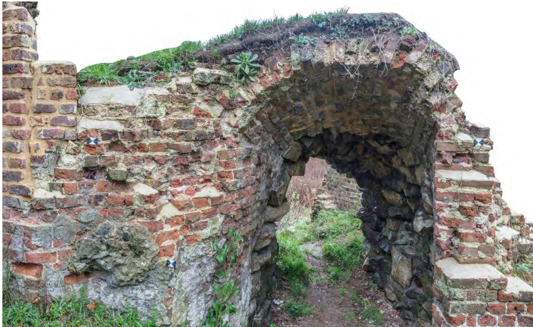
Figure 15: Rectified photography of a section of the Grotto, showing the variety of different repairs
