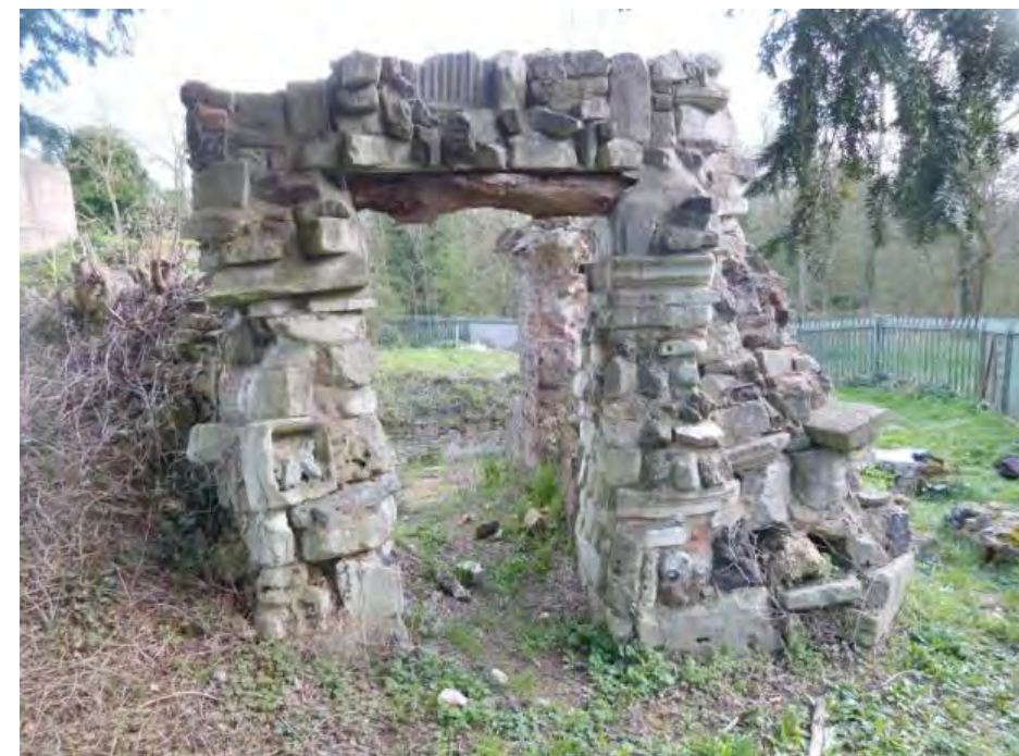
Fig 7: west elevation of Zone B – note voids in buttress on the right
