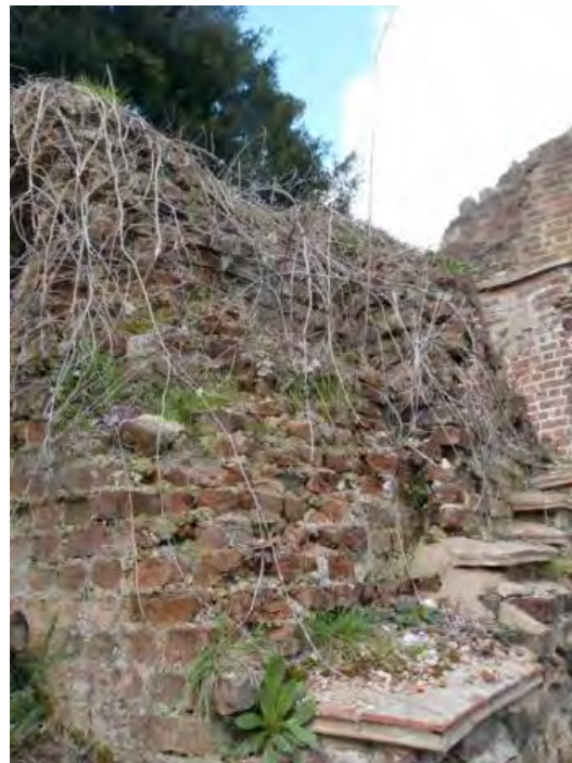
Fig 28: detail of brickwork showing separation of front face due to root growth
