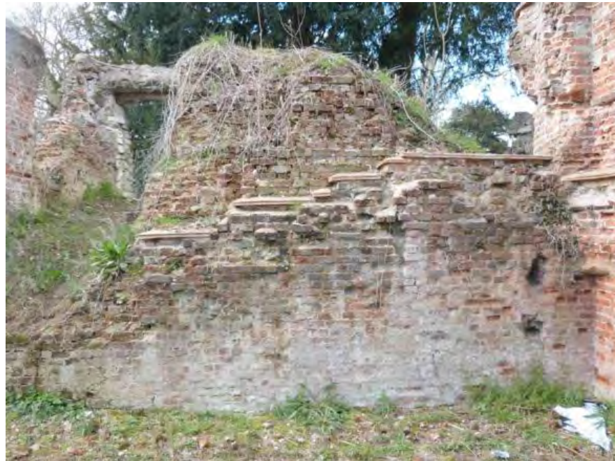
Fig 27: Zone L with tile creasing
