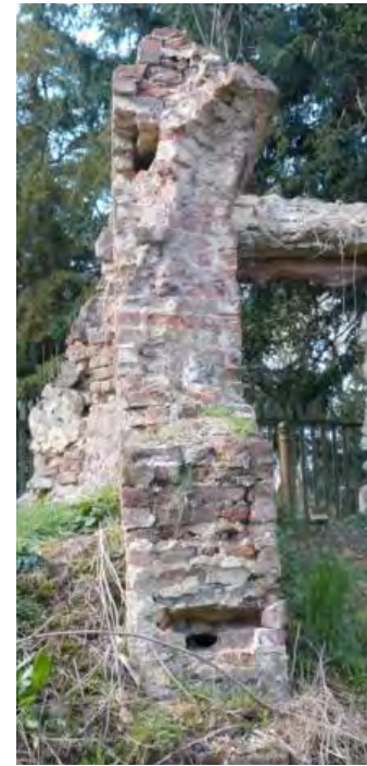
Fig 5: east elevation of zone A of showing voids and loose bricks
