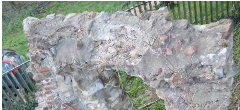
Fig 8: detail of top of wall showing decayed mortar capping
