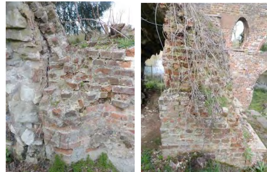
Fig 10: Zone C – east jamb of door showing void Fig 11: Zone C – east section
