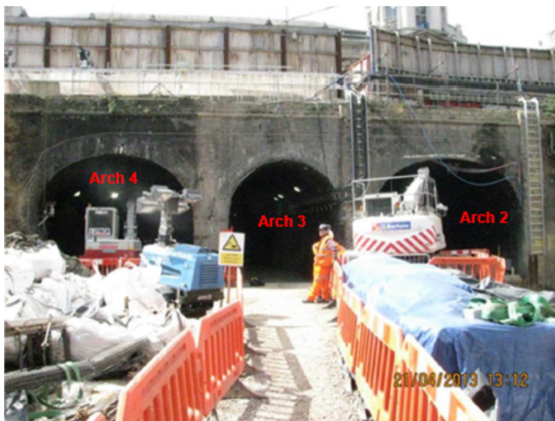
Plate 2 View of East Elevation of Lindsey Street Bridge (looking west).
