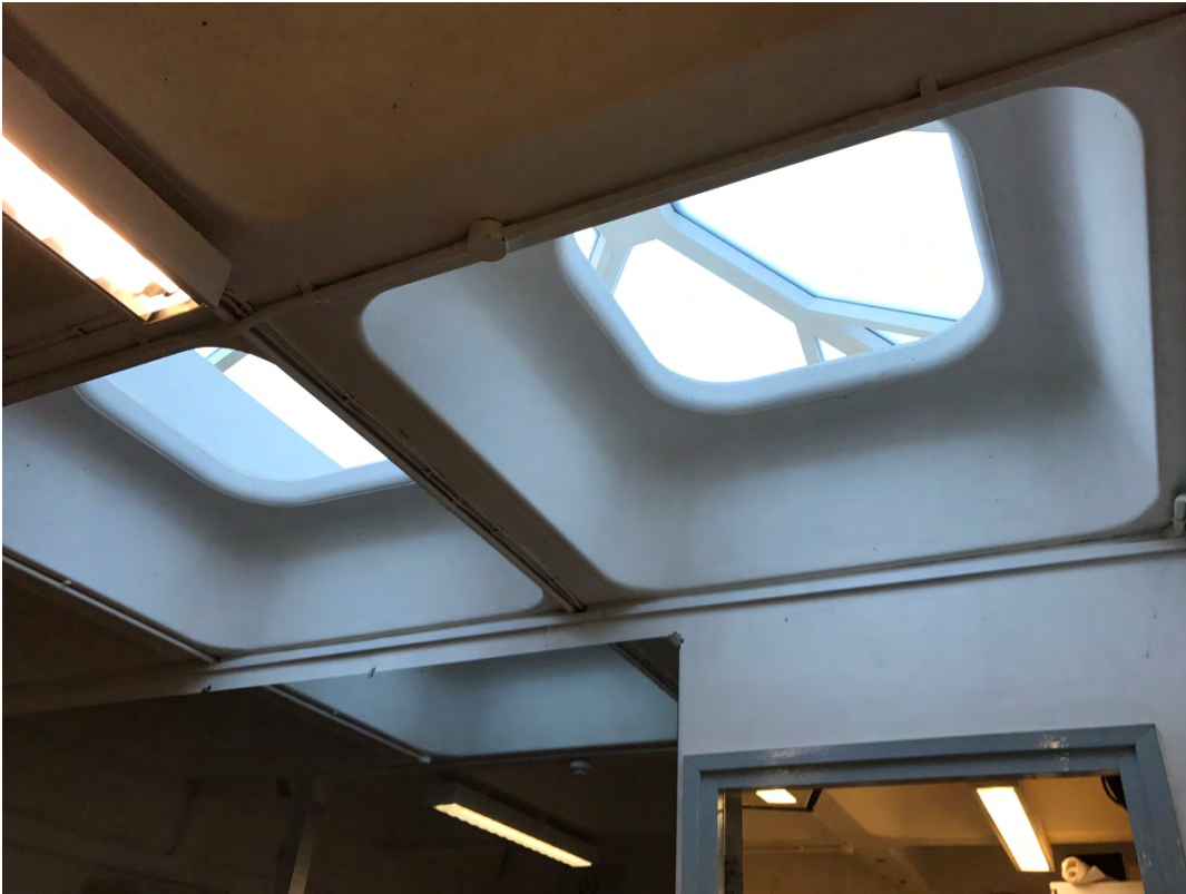
View of replacement rooflights from within staff office
