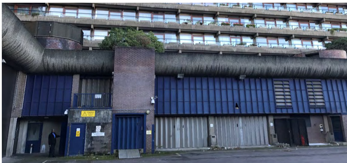
The delivery yard, with paneled façade. Breton House is above the podium level.
