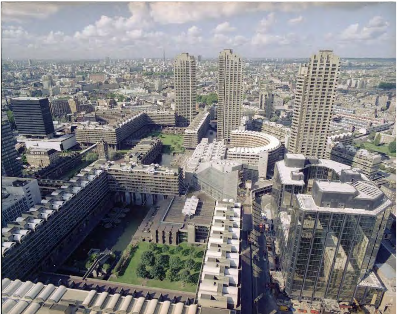
Overview of the Barbican Arts Centre in its context
