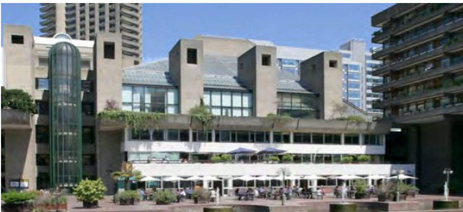
Lakeside façade recesses should remain unenclosed, and upper level planters maintained
