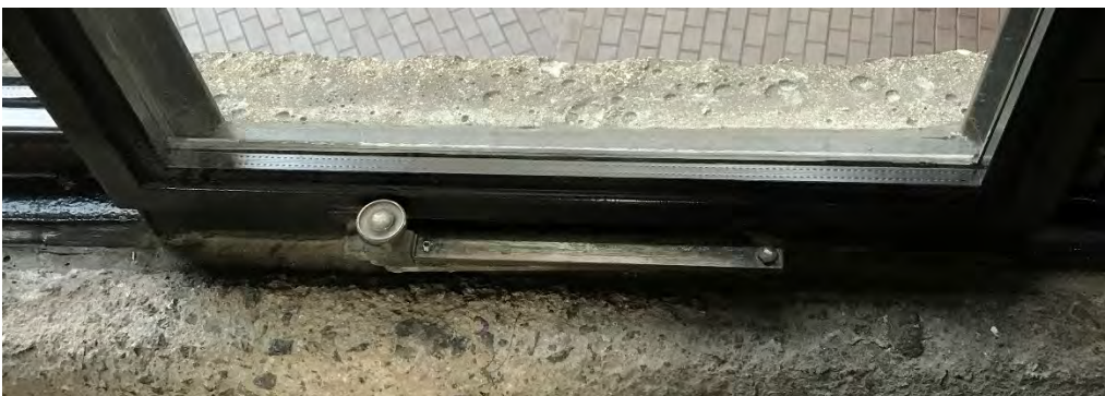
Window detail with new double glazing
