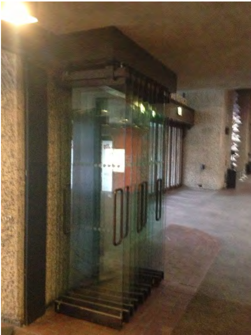
Retractable doors to lift hall
