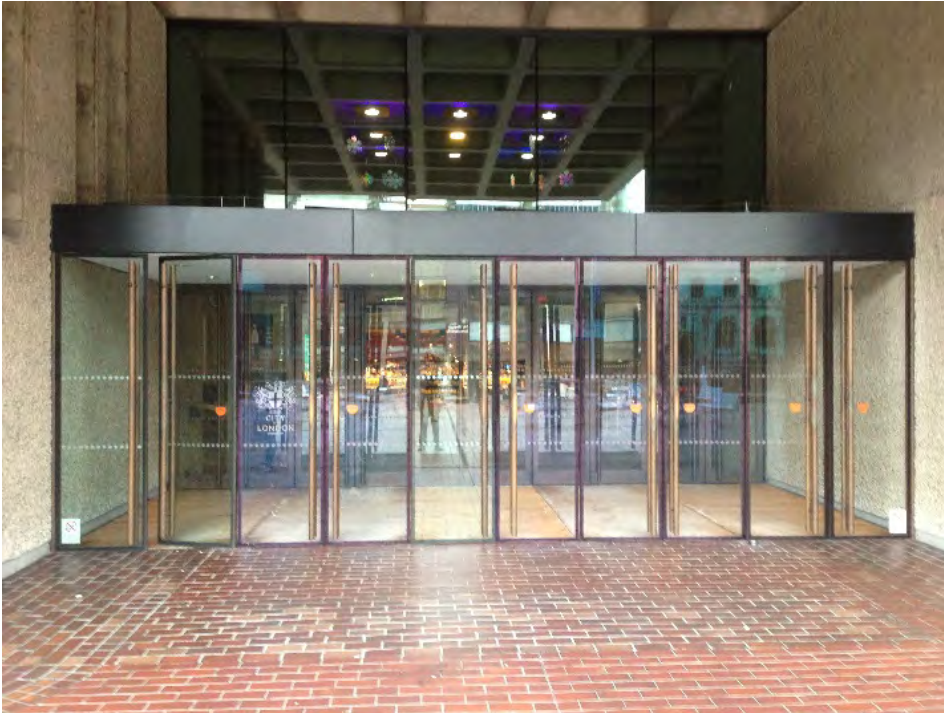
New lobby addition on south façade
