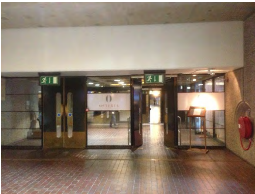
Looking east towards outer lobby (Level 2)
