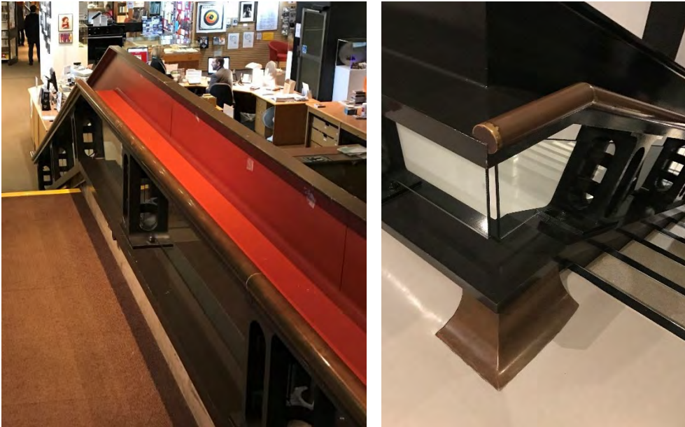
The unique Barbican guarding shelf section, a guiding presence throughout the Arts Centre
