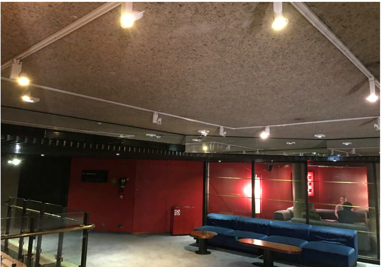
Upper foyer showing inserted glazed screen and additional face fixed track lighting.
