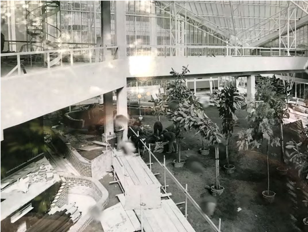
The Conservatory under construction
