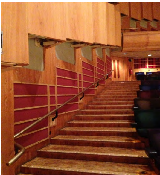
Details of new adjustable acoustic panels and new acoustic linings on side and rear walls
