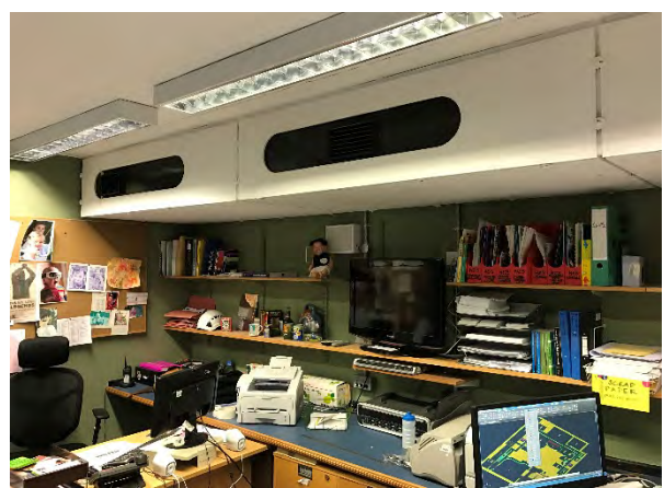
Original oval slotted duct detail
