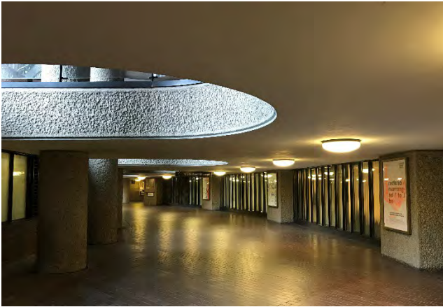
Offices surrounding Frobisher Crescent walkway, showing original close mullioned façade screen
