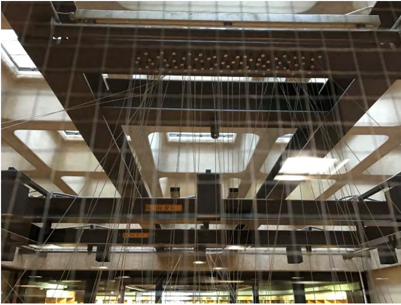
The gantry apparatus fixed below principal foyer rooflight
