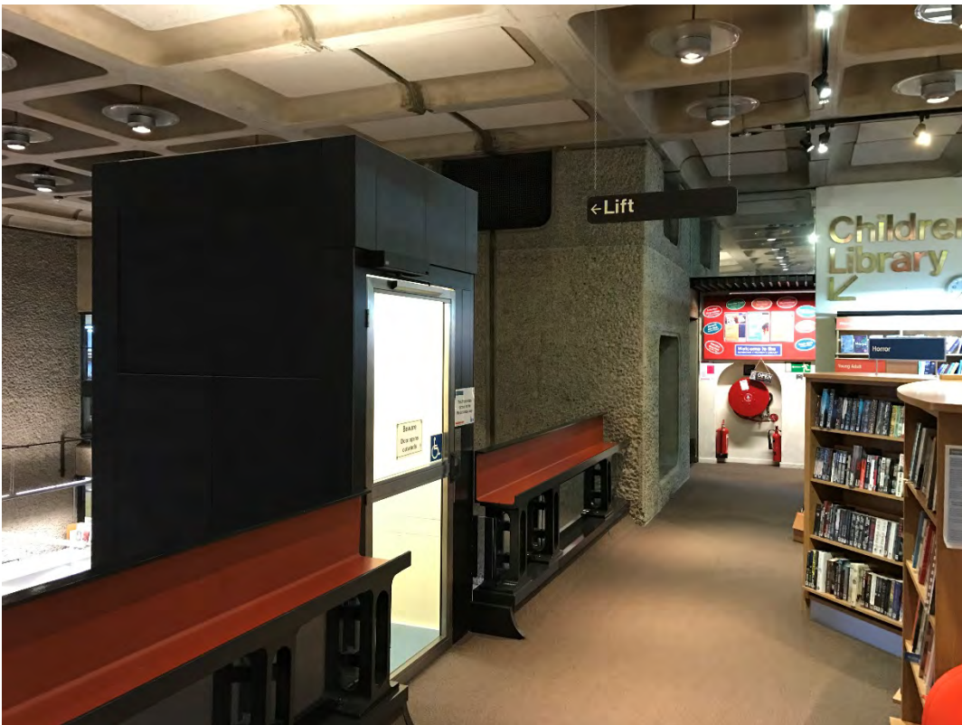
The lift connecting the two Library floors. Note consistent use of guarding detail.
