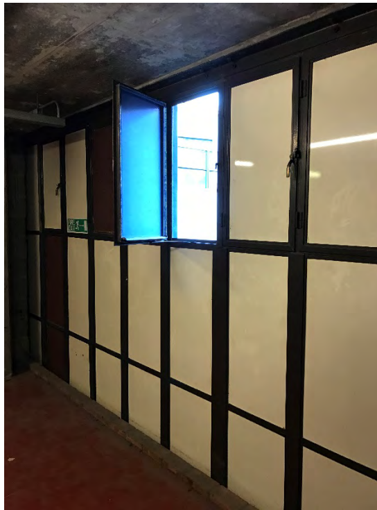
Inside view of panelling on external façade
