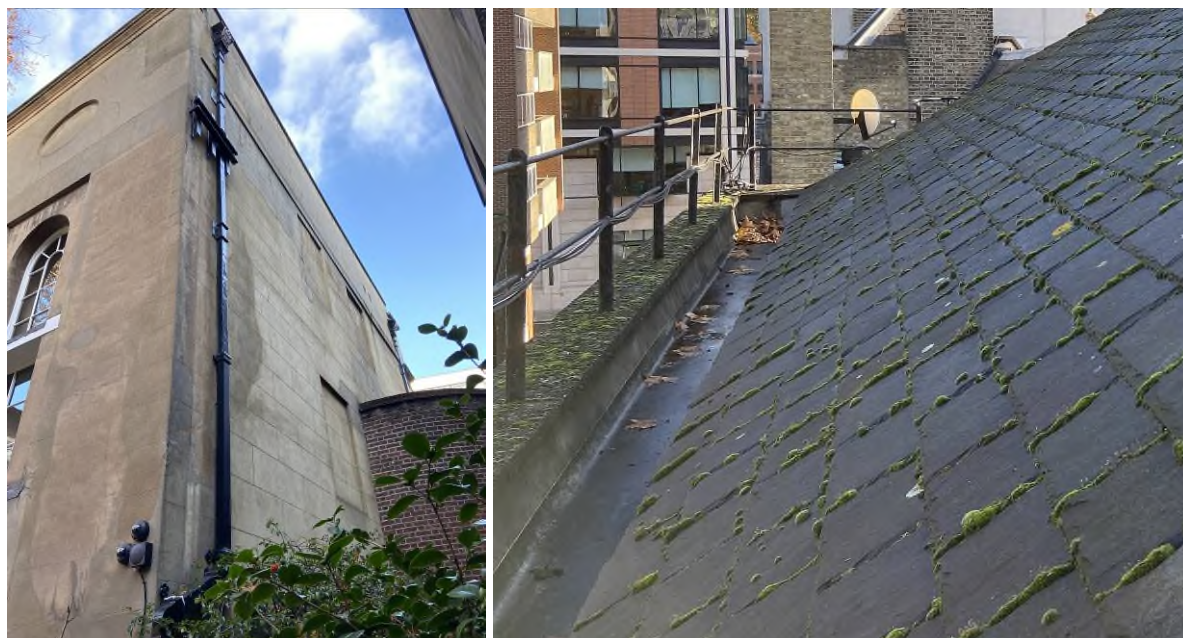
Figures 39 & 40. Details of the roof, parapet gutter and downpipe on the Great Hall.
