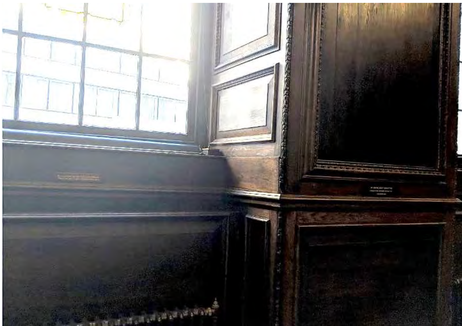
Figure 14: Correct arrangement of internal sill, east side of Hall
