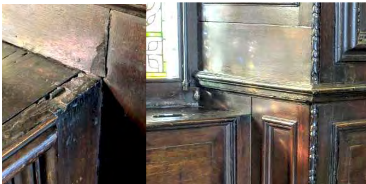
Figure 13: Missing internal sill boxing beneath the Cranmer window. Trimmed panel rail with section through mortice/tenon clearly visible.
