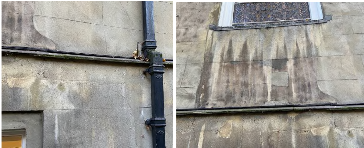
Figures 21 & 22. Details of cracking to the render and previous repairs on the west elevation of the Great Hall.
