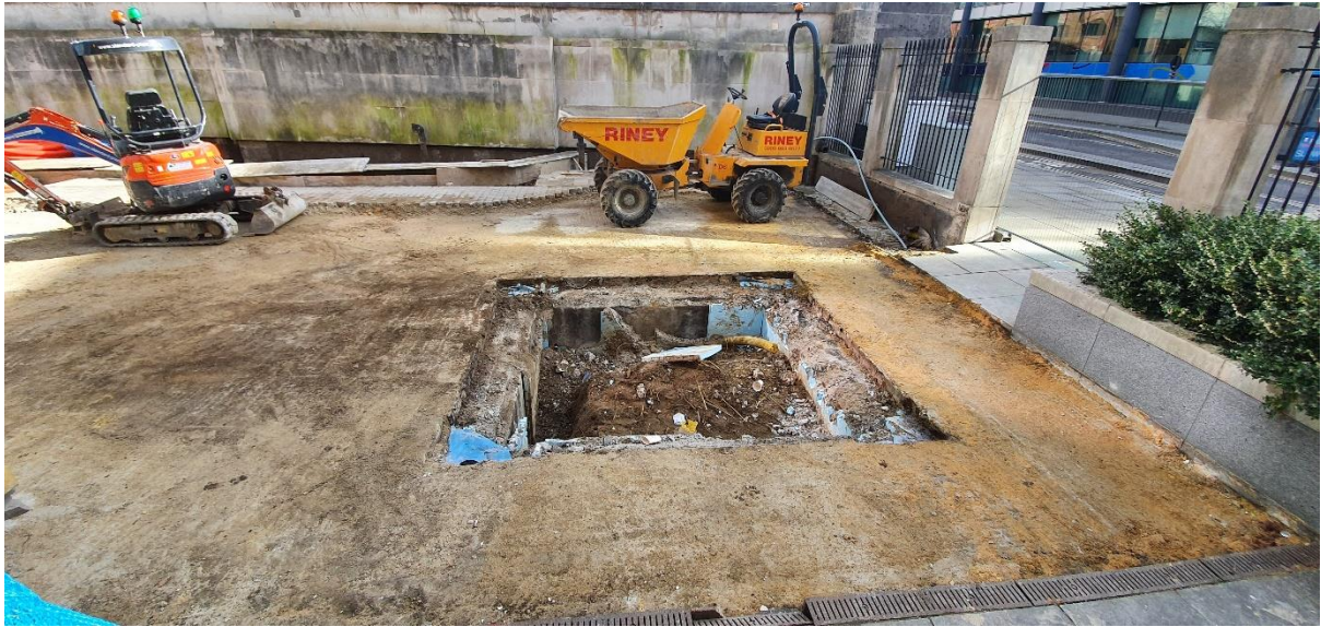
Photo of restrictive cavern for tree created during construction of Old Change House
