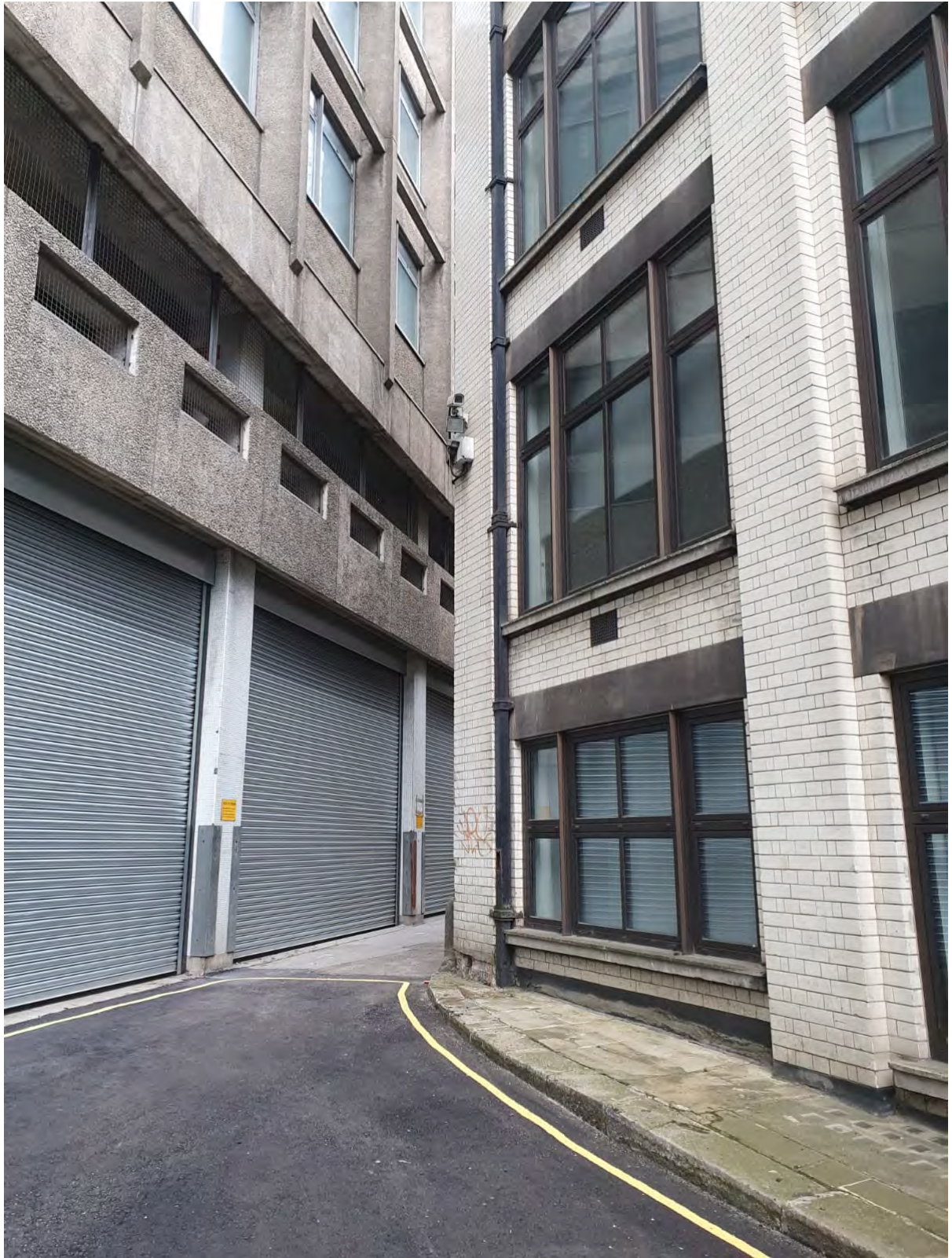
Image 17: Corner of Turnagain Lane
