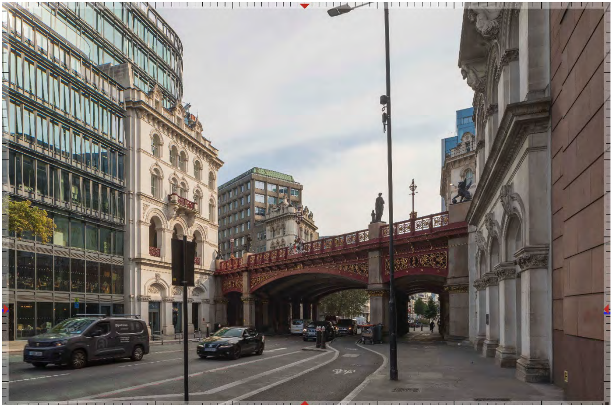
Image 2: View of site from north of Holborn Viaduct bridge.
