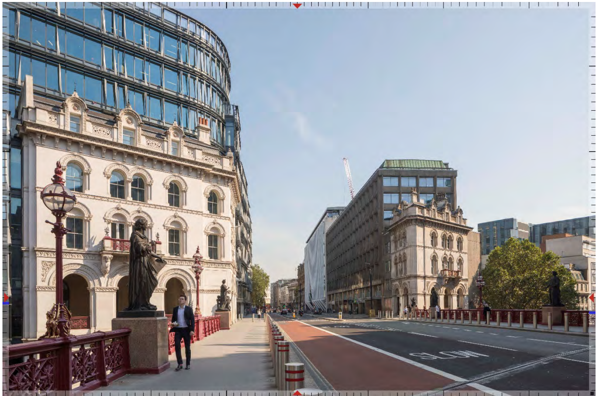
Image 6: View of site looking east from Holborn Viaduct bridge
