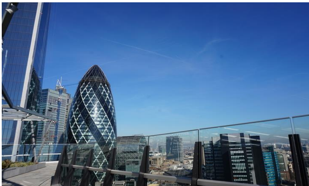
Balustrade on roof terrace at 120 Fenchurch Street
