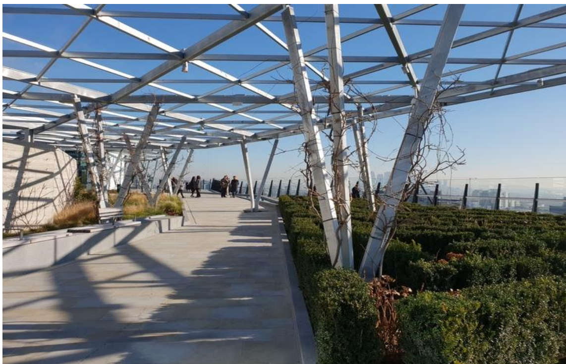
Planting on roof terrace at 120 Fenchurch Street
