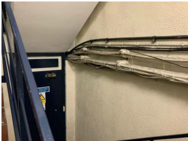
Figure 20: Service not related to firefighting shaft passing through the firefighting stair
