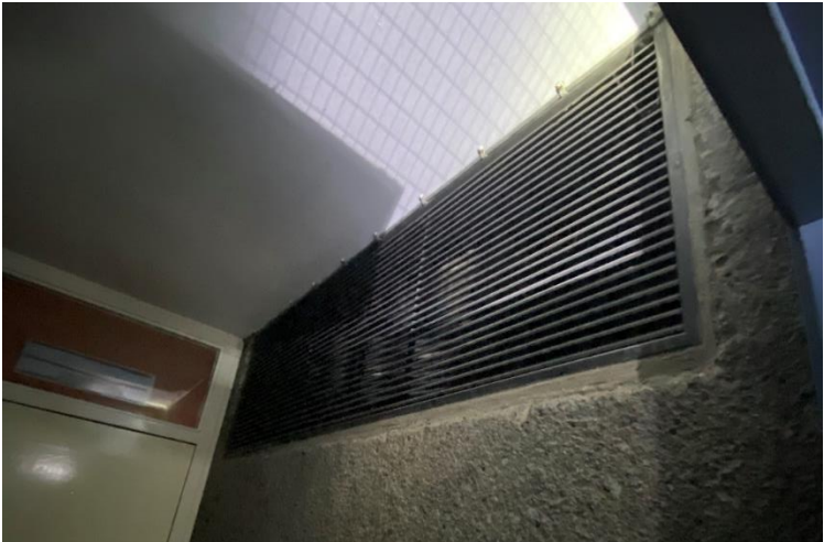
Figure 12: Louvre connecting the small lobby and the electrical riser
