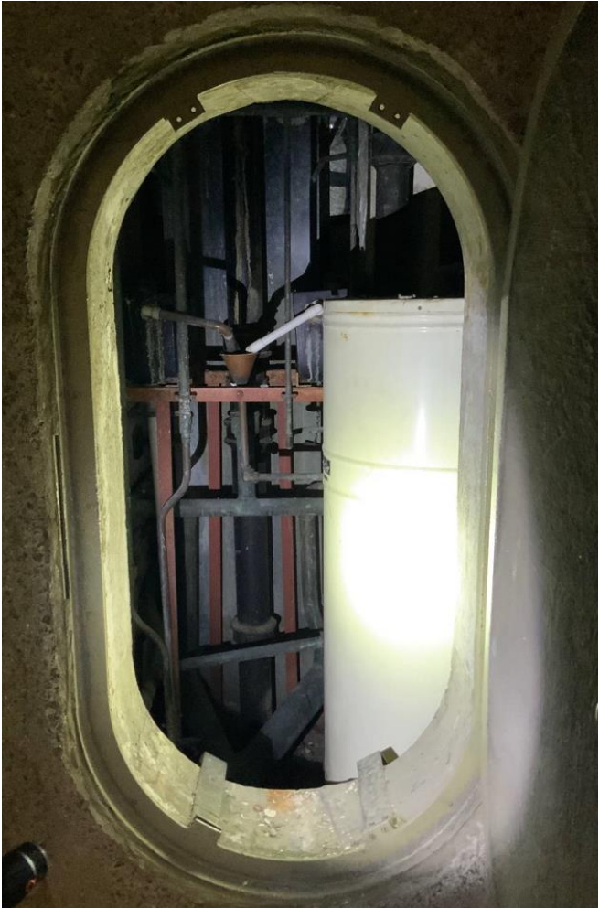
Figure 15: Risers within the lift lobbies
