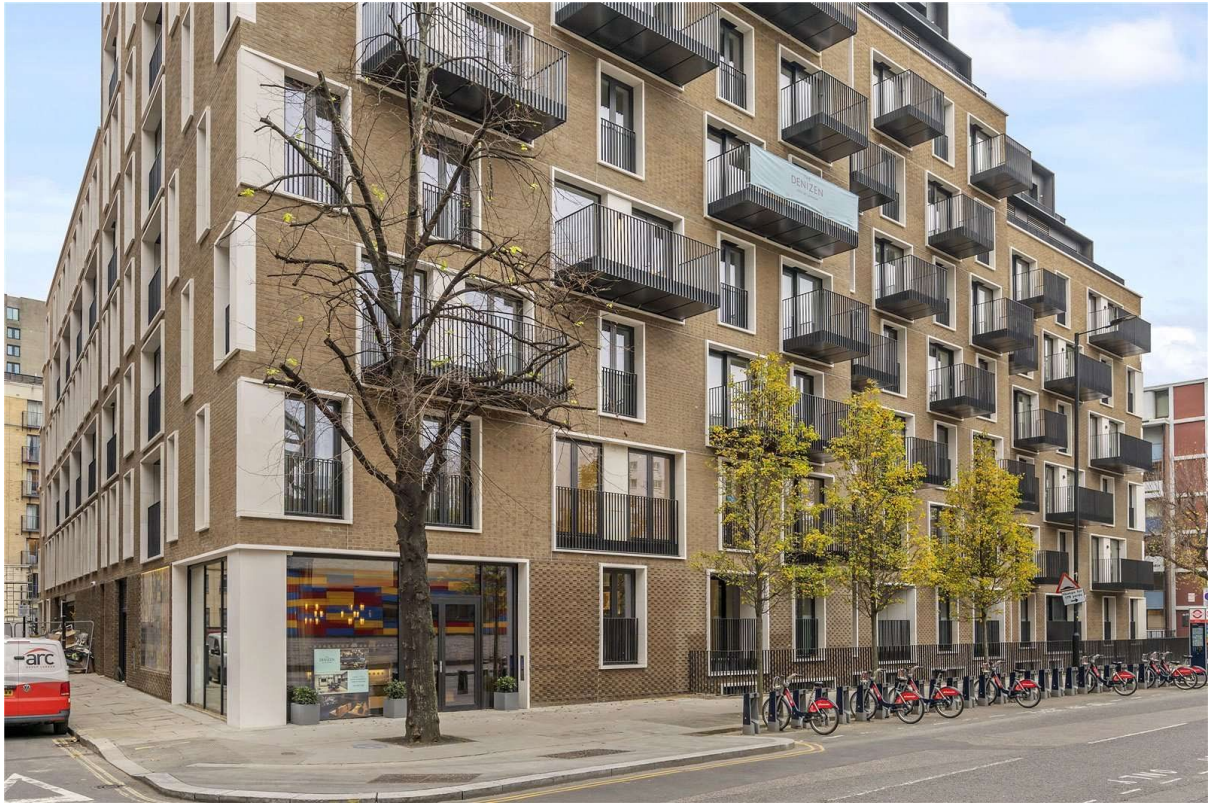
Before: Golden Lane looking north-west
