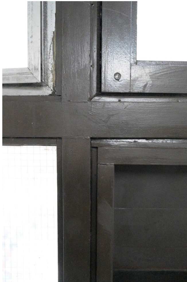
Image 11 – typical profiling of Goswell Road window frames
