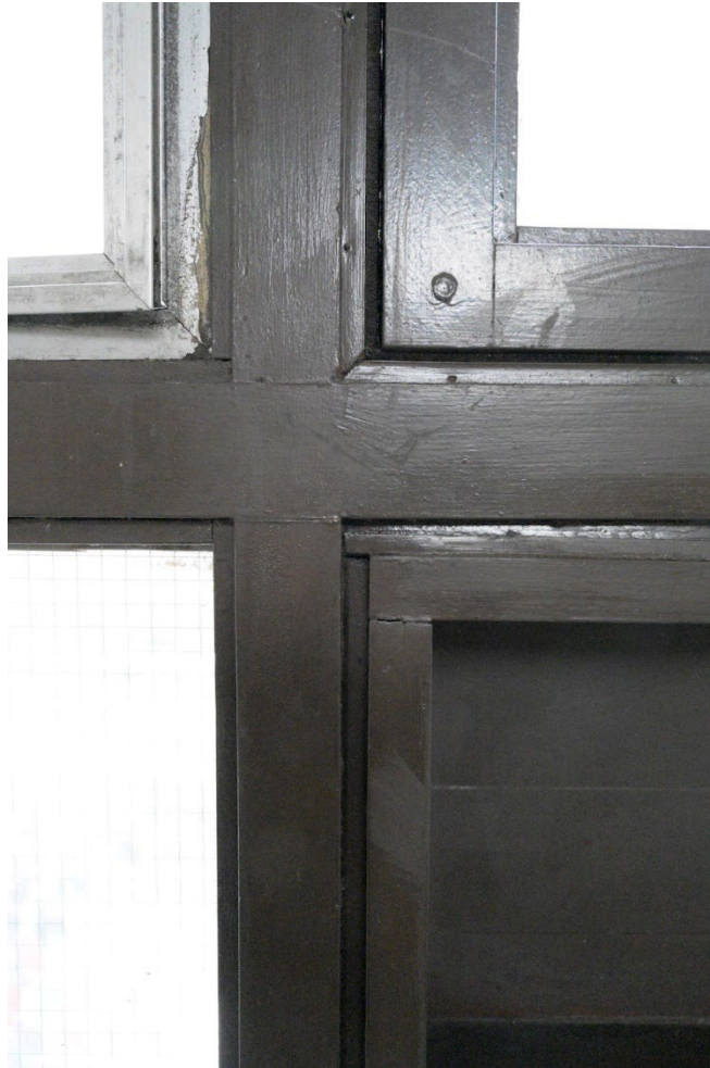
Image 11 – typical profiling of Goswell Road window frames
