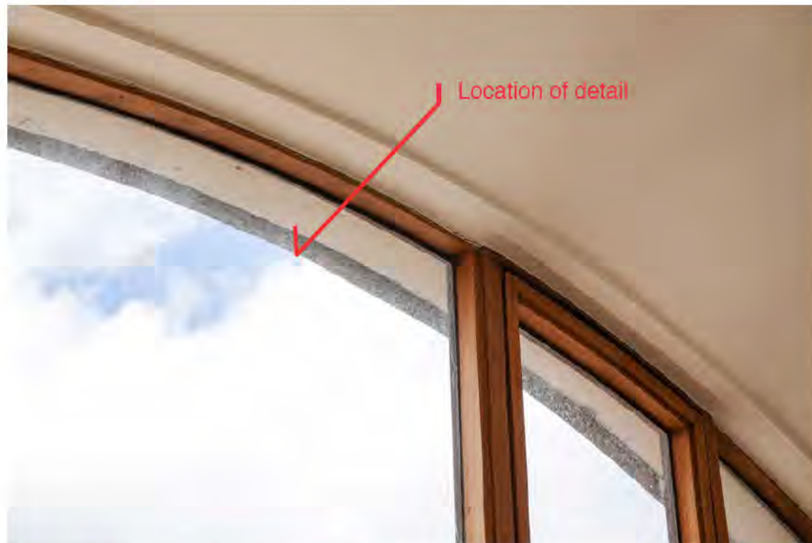
PHOTO OF EXISTING CONDITION
