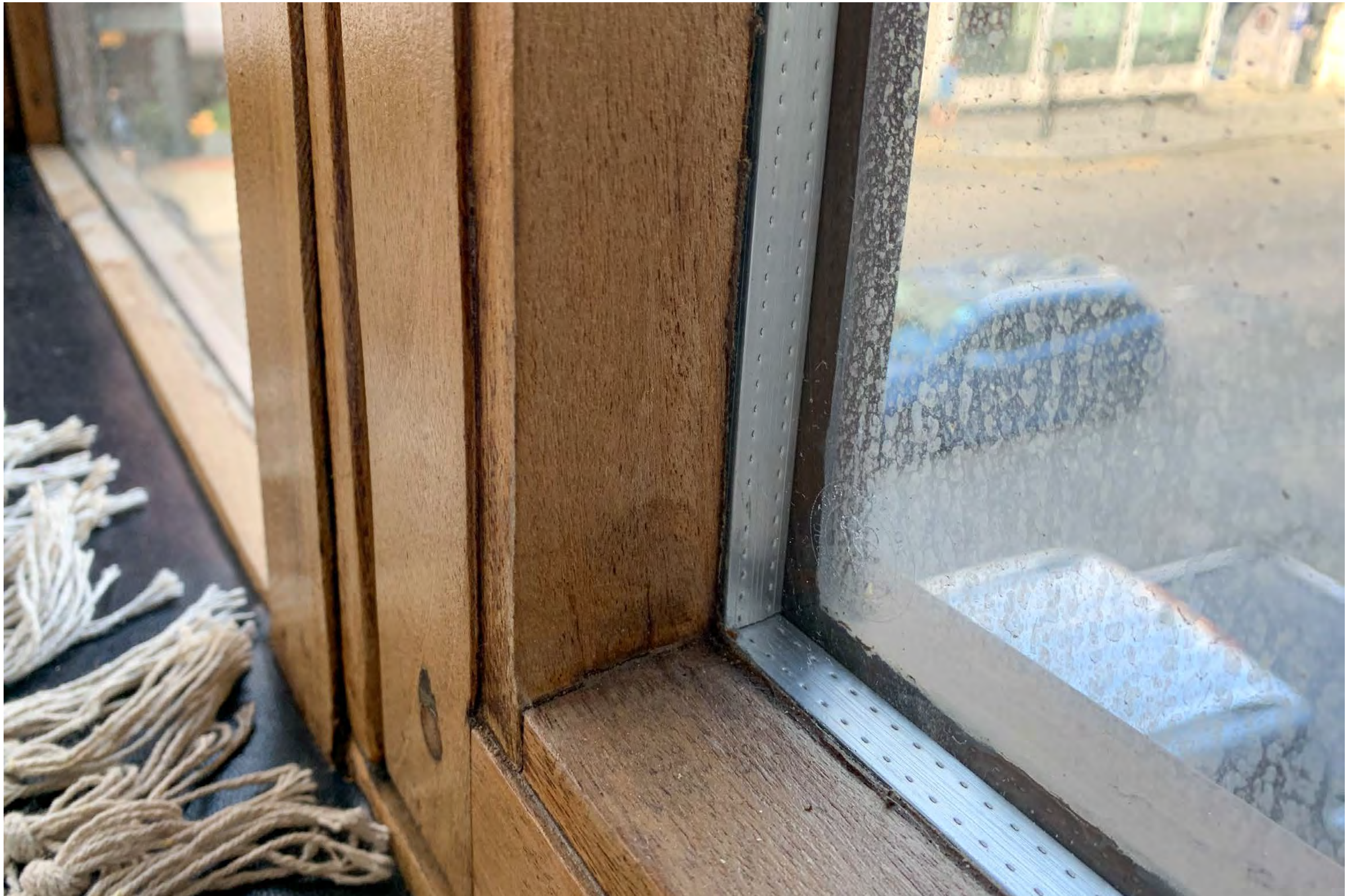
EXAMPLE OF DOUBLE GLAZING IN EXISTING FRAME
