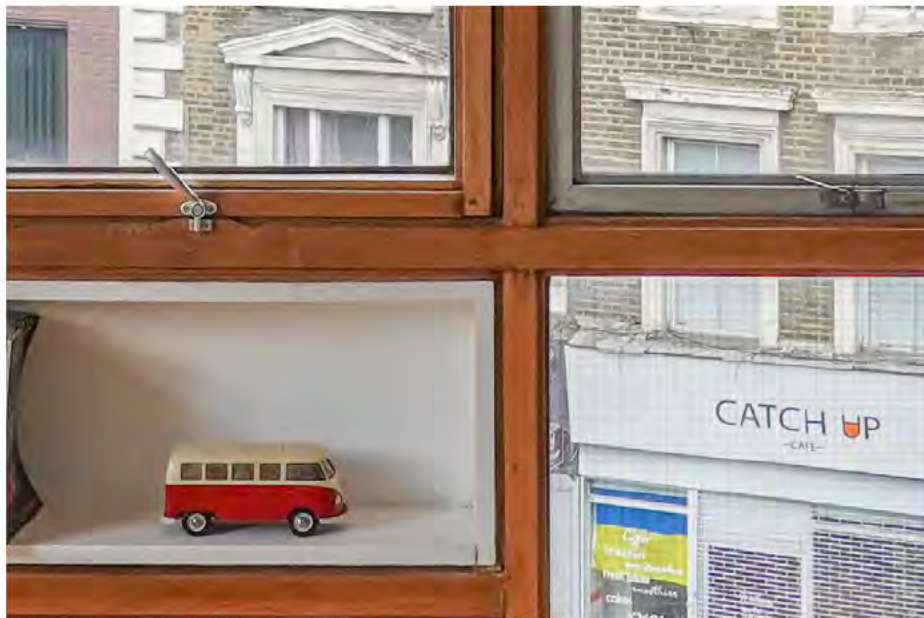
Photo showing EXISTING junction
