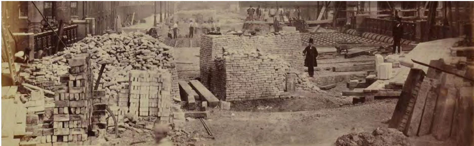
Fig. 56: Setts waiting to be laid, Holborn Viaduct, 1869 (London Picture Archive)
