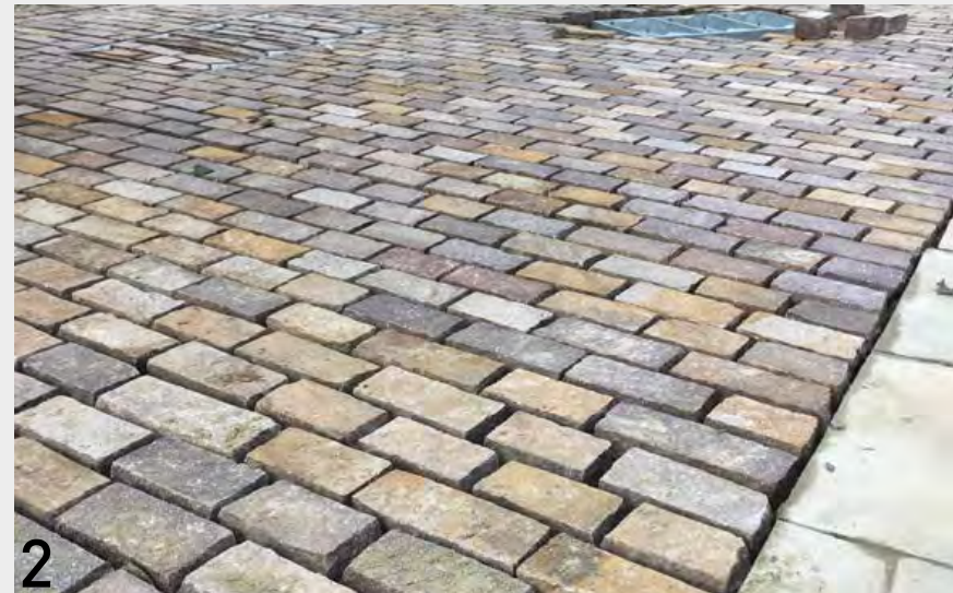
2 Setts are laid to tessellate with each other which can be time consuming
