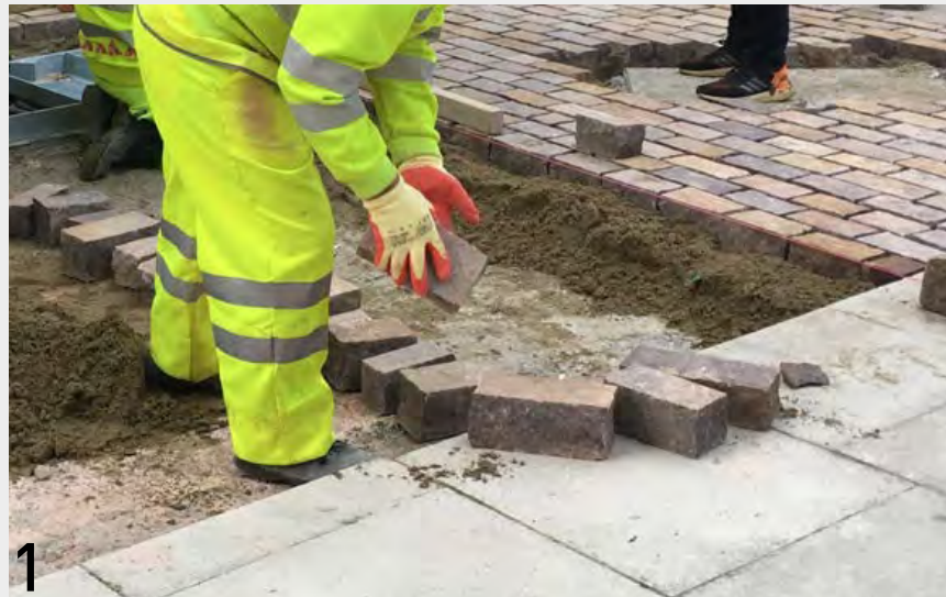
1 Setts are individually selected and laid on a specially prepared sandy bed
