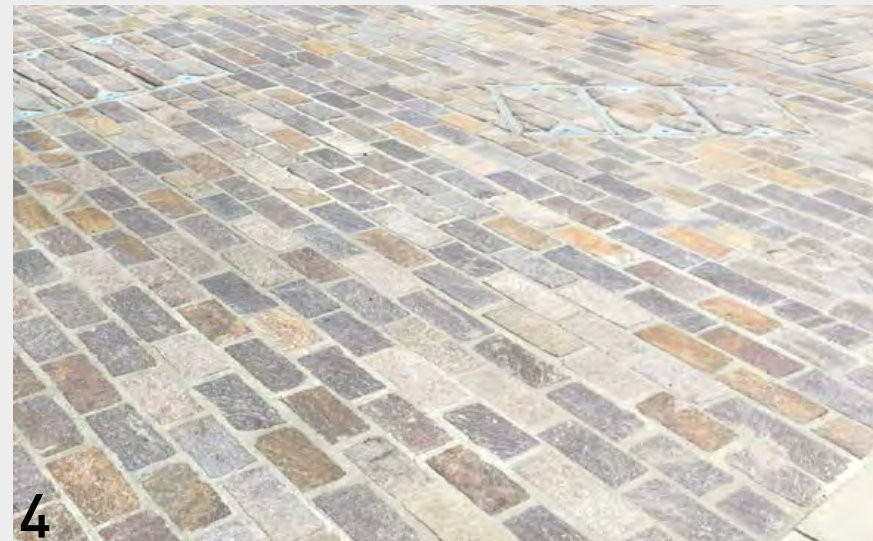
4 If the work is good, the finished result should have a relatively even surface
