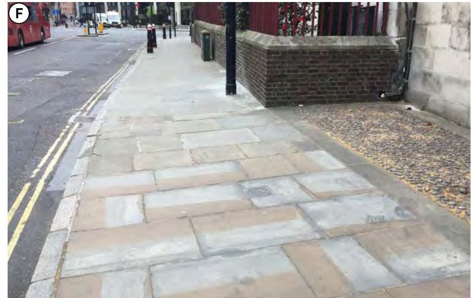
Fig. 34: Three different types of York Stone paving present at the southern end of Giltspur Street (Location F on Fig. 29 )
