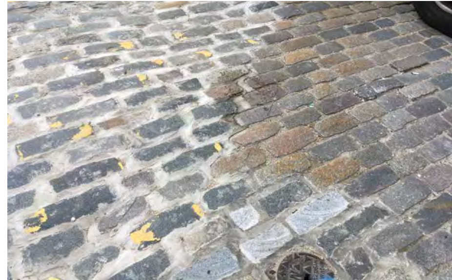
Fig. 58: The same location after setts are re-laid
