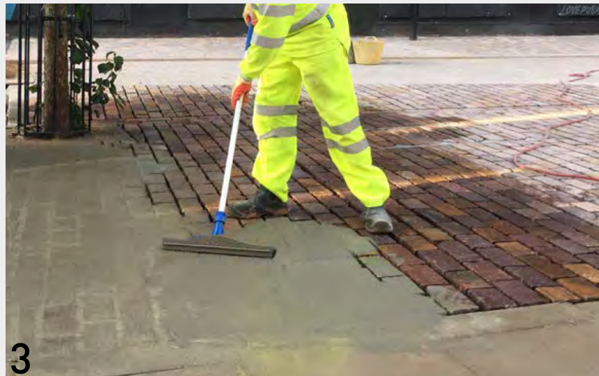
3 Once setts are laid, a grout mixture is poured on top and brushed over
