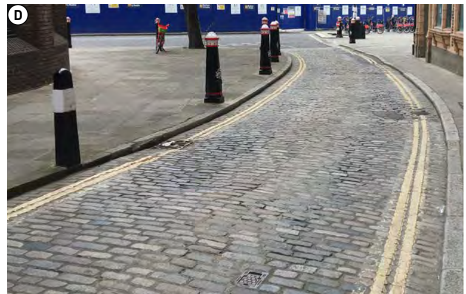
Fig. 30: Historic granite setts on Cock Lane (Location D on Fig. 27 )
