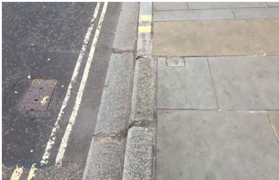
Fig. 35: Granite kerbstones of different widths
