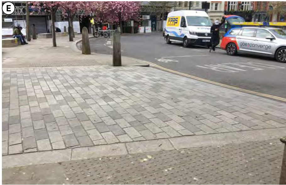
Fig. 32: More modern granite setts, West Smithfield (Location E on Fig. 27 )
