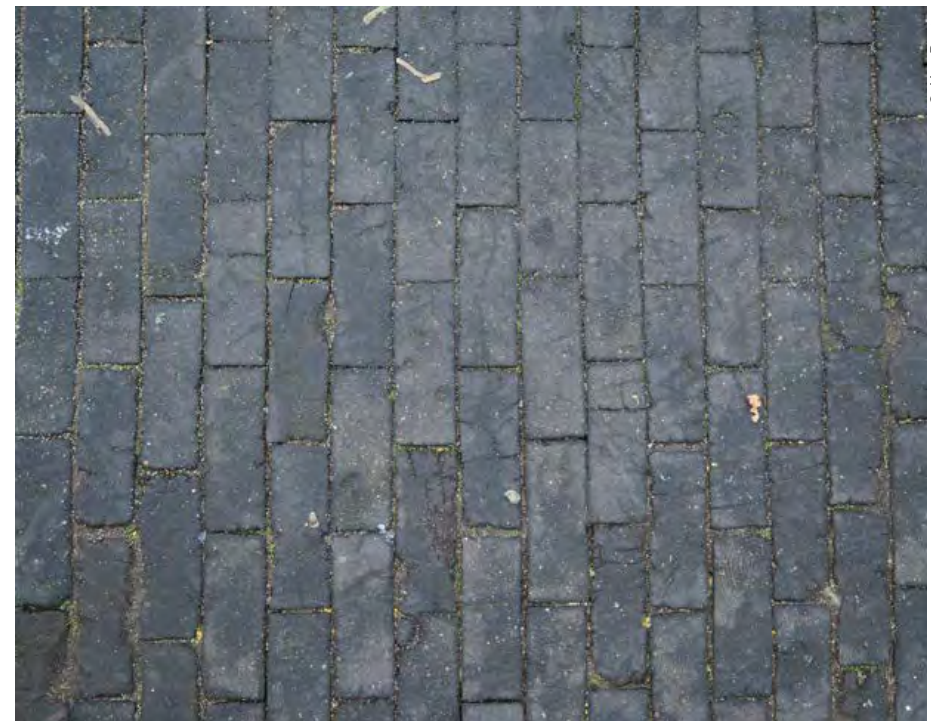
Fig. 22: Wooden blocks on Chequer Street (2021)
