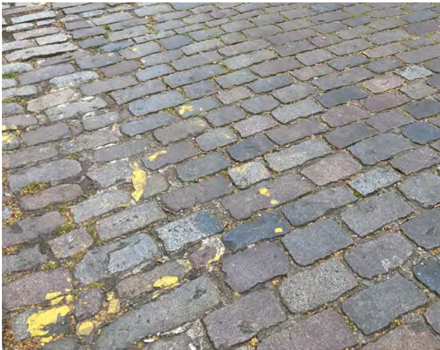
Fig. 21: Granite setts dating to the 1860s (with potentially earlier examples), Charterhouse Square (2021)
