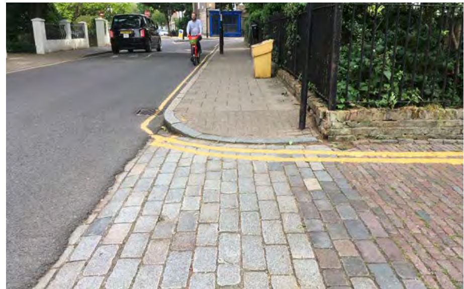
Fig. 61: Setts in the foreground are larger than those (right) on the less trafficked route (Thornhill Road, Islington)
