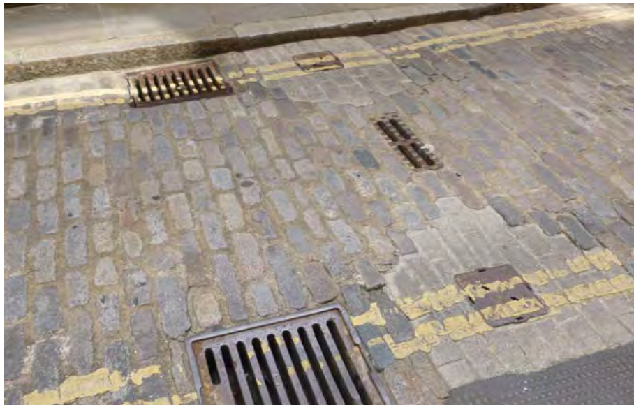
Fig. 37: Different elements (including drain and man hole covers) set within the road and pavement of Cock Lane
