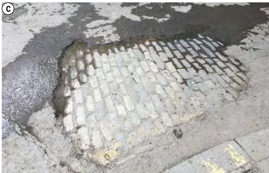
Fig. 29: Granite setts hidden under later asphalt surfacing (Location C on Fig. 27 )
