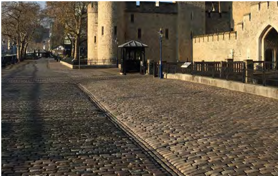
Fig. 64: Drainage gully (Tower Wharf, City of London)
