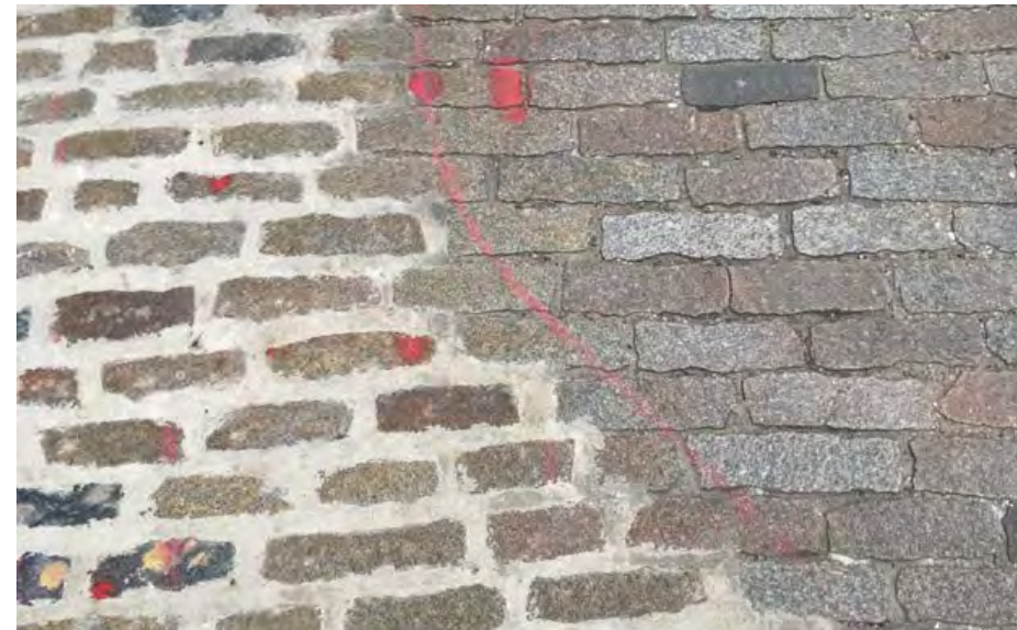
Fig. 59: The special qualities of setted surfaces are vulnerable to repeated relaying
