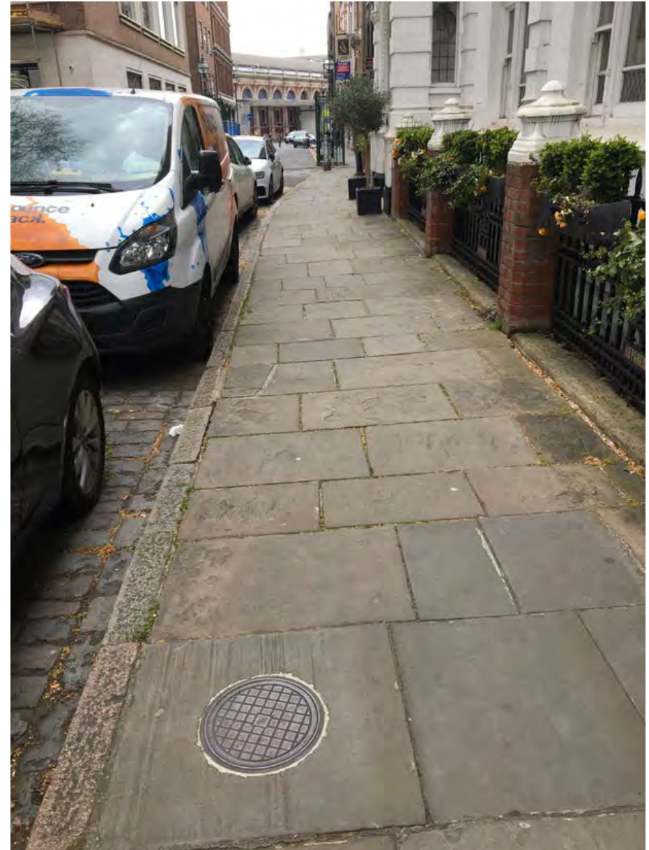
Fig. 24: York stone paving with granite kerbs dating to the 1860s, Charterhouse Square (2021)
