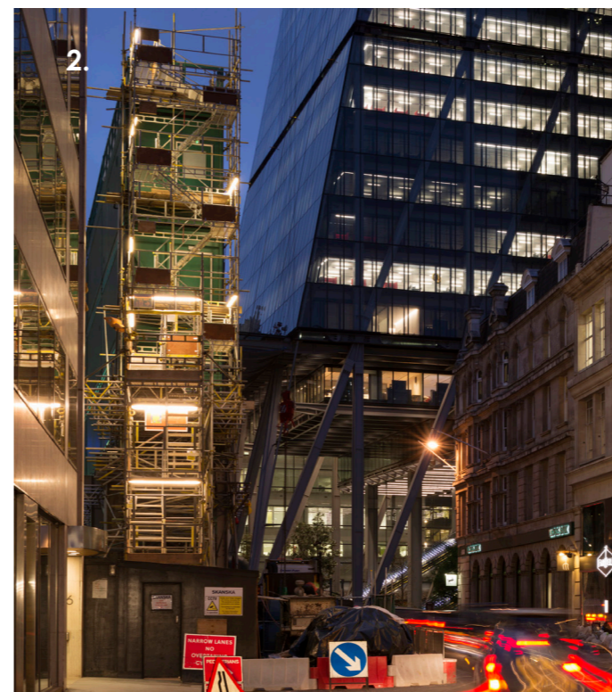
2. Temporary construction lighting can cause glare, light spill and light pollution. Photography by James Newton.
