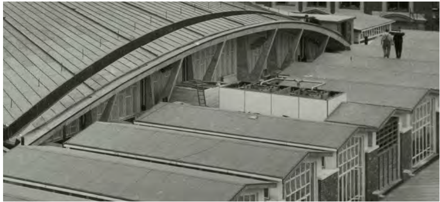
Archive photograph of East Poultry Avenue original roofscape showing precedent plant detail to monitor roof
