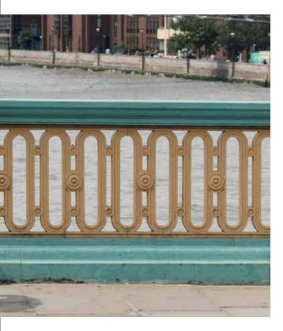
and white colour scheme will be restored, and the rust staining removed. The benefits of this project will be visibly apparent over the coming years as the refurbishment traverses the bridge, span by span.
